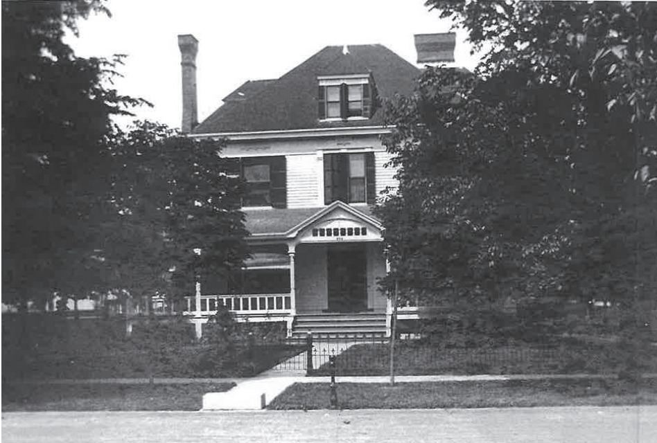
Original Marion Street View prior to 1929
