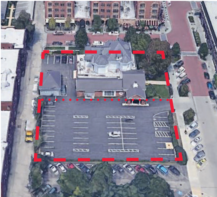
Aerial View - The red dotted line in middle of property indicates the location of a subdivided lot for a single family residence and adjacent development parcel. If house is restored to original design, only 50% of the property would be available for redevelopment.
