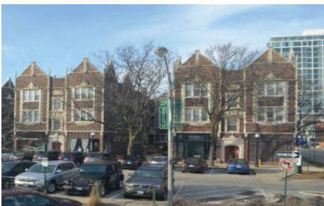
Courtyards with active street level
