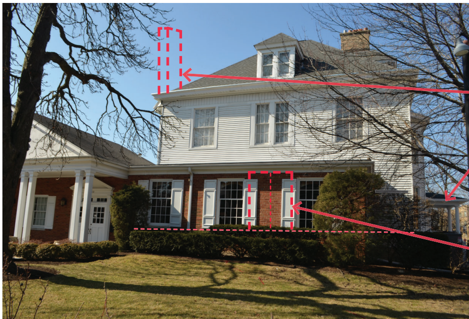
Existing Marion Street View of Funeral Home
