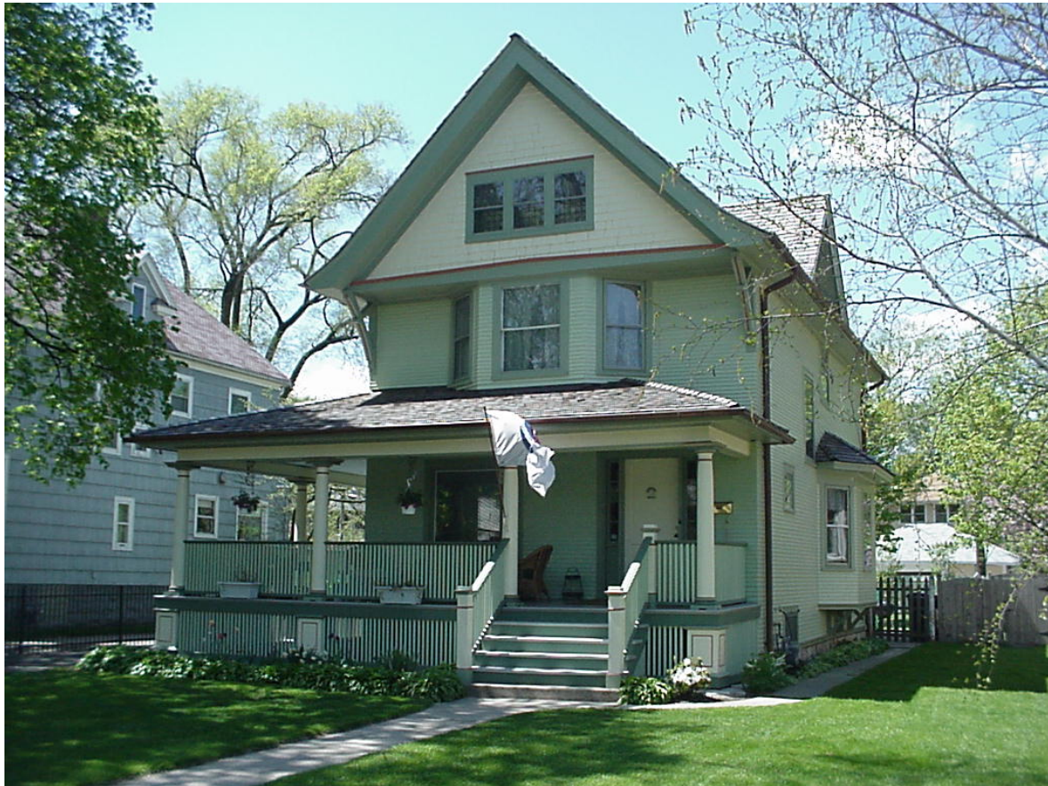
643 N. Oak Park Avenue (FIRE RESTORATION) Bill Bango and Lori Malinski
