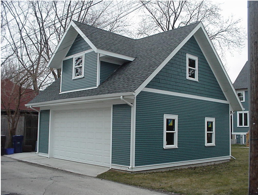
163 N. Ridgeland Avenue (RESTORATION, NEW GARAGE CONSTRUCTION) Charles Moelter Gus Kostopulos, Architect
