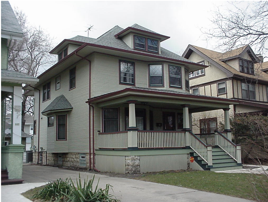
525 S. Elmwood Avenue (RESTORATION, REHABILITATION, ADDITION) S. T. Gunderson & Sons, 1909 Mike and Karen Iannaccone Magner & Manalang Architects Kevlar Construction Inc.
