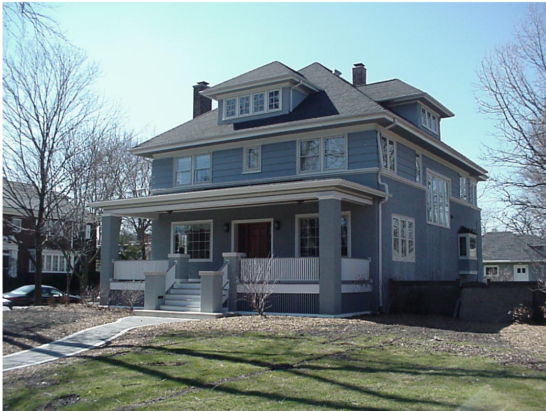
403 N. Scoville Avenue (FRONT PORCH ADDITION) A. Zwycke House, 1909 Jay and Betsy Tharp Sher-Bergstrom Architects A. J. Madden & Sons
