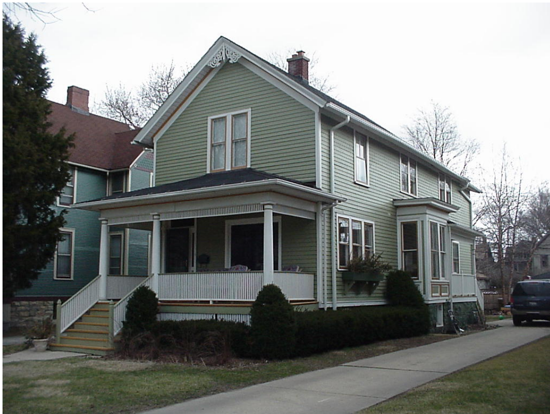
244 Clinton Avenue (RESTORATION) c. 1903 Ken Javor Construction
