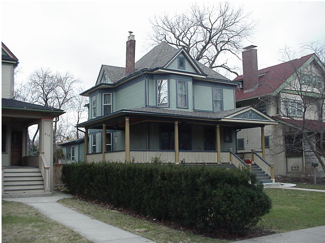
209 S. Scoville Avenue (RESTORATION, ADDITION)
