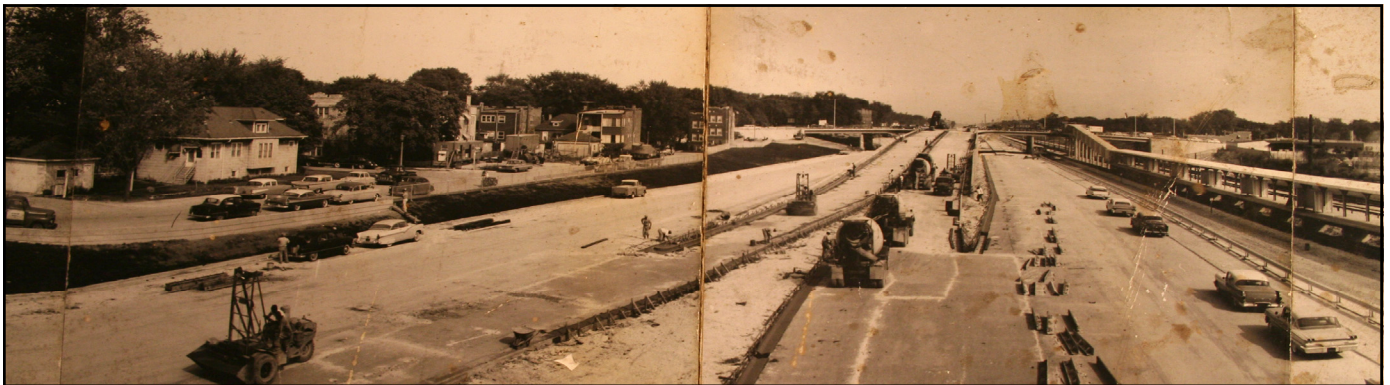
Figure 9: View of center lane exit ramp under construction (ca 1956). Images courtesy of the Historical Society of Oak Park and River Forest
