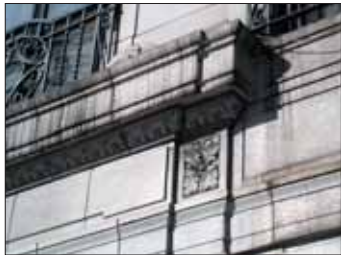
facade detail UIC photo
