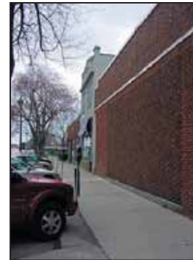
blank facades on Harrison Street need improvement UIC photo
