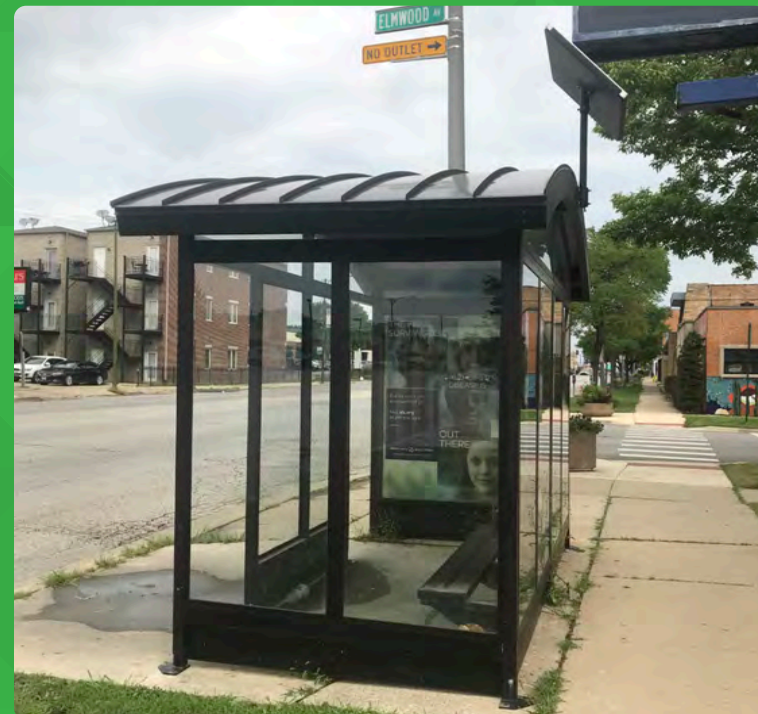
▶ Near-side eastbound bus stop with a shelter North Avenue at Elmwood Avenue – Oak Park, IL Photo credit: Kimley-Horn
