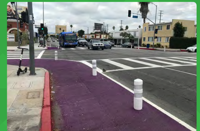
▶ Pilot curb extension Pico Blvd / Hauser Blvd – Los Angeles, CA Photo credit: Kimley-Horn
