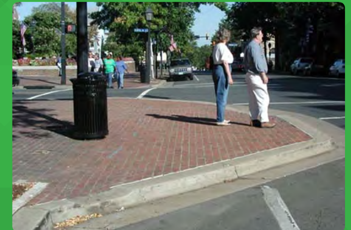
▶ Corner curb extension Photo credit: Alexandria, VA
