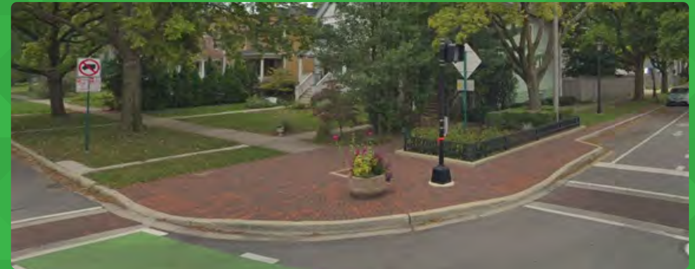
▶ Corner curb extension on one side with on-street parking Chicago Avenue / Harvey Avenue – Oak Park, IL Photo credit: Google Streetview
