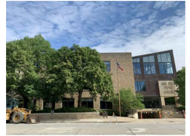
3. LOOKING NORTH TO OAK PARK PUBLIC LIBRARY
