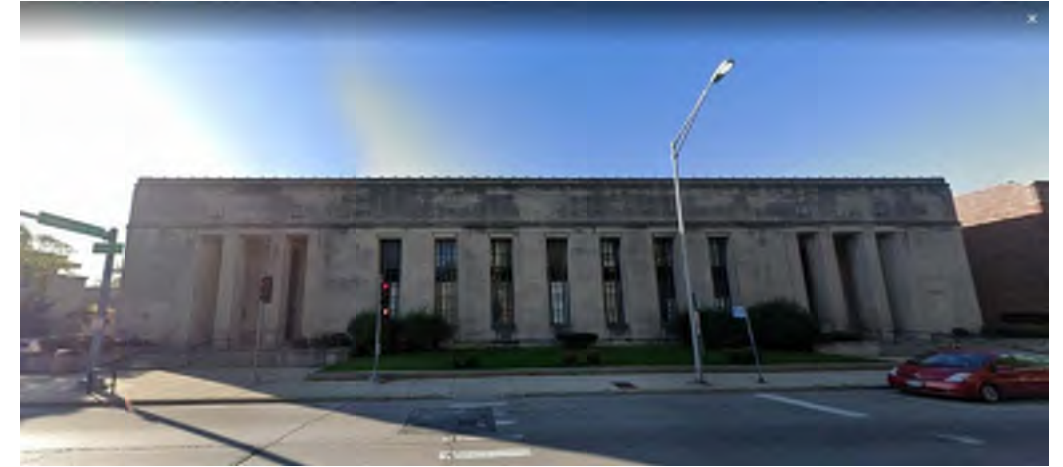
3. LOOKING SOUTH TO U.S. POST OFFICE BUILDING (901 LAKE STREET)
