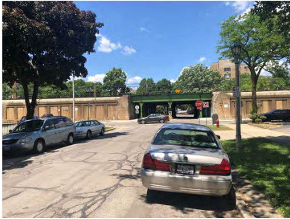
Looking north along Kenilworth Ave at South Blvd
