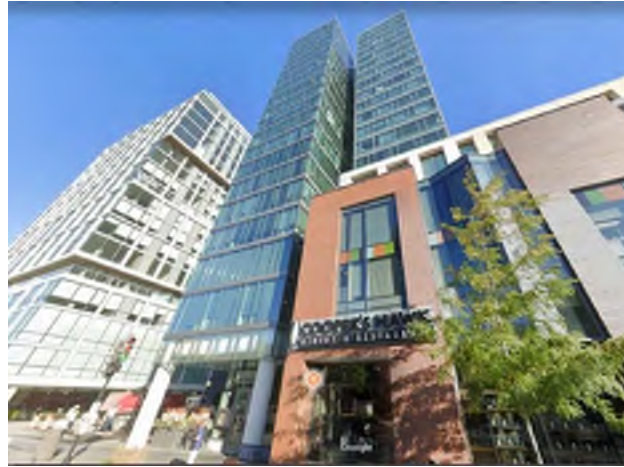
1. LOOKING NORTH TO 950 LAKE STREET
