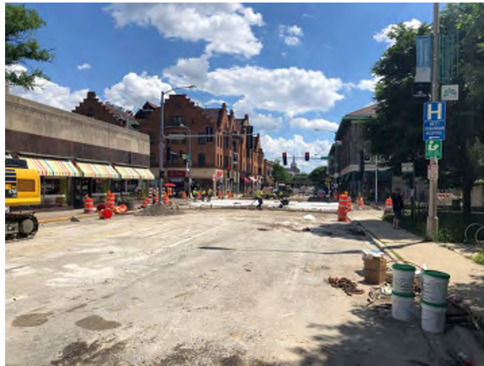
Looking south along Oak Park Ave at Lake St
