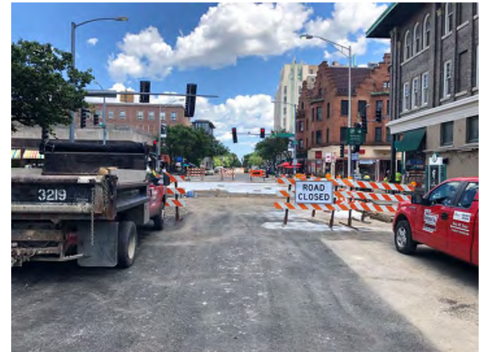
Looking east along Lake St at Oak Park Ave
