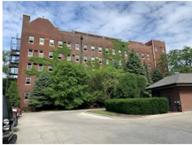
1. VIEW WEST FROM SITE TO 855 LAKE
