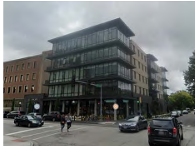
5. LOOKING NORTH TO 702 LAKE STREET
