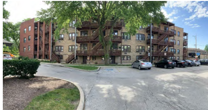
5. VIEW EAST FROM SITE TO 815 LAKE
