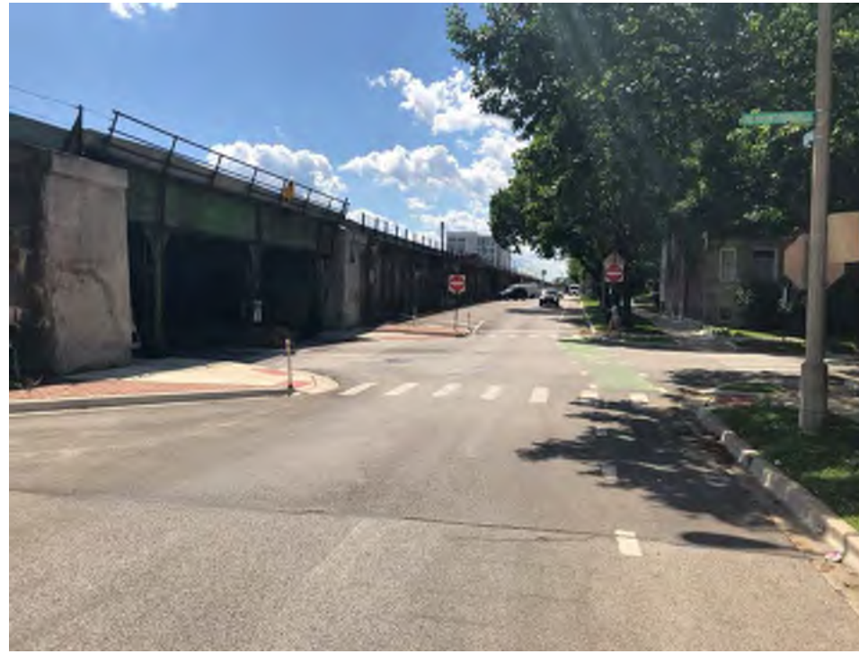
Looking west along North Blvd at Kenilworth Ave
