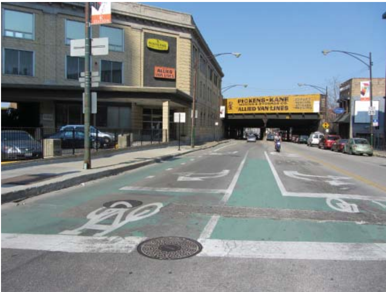
NEIGHBORHOOD GREENWAYS PAVEMENT MARKING WITH TURN ARROW Are used where Neighborhood Greenways are offset, jog, or where two Neighborhood Greenways intersect. Photo credit: J. Maus
