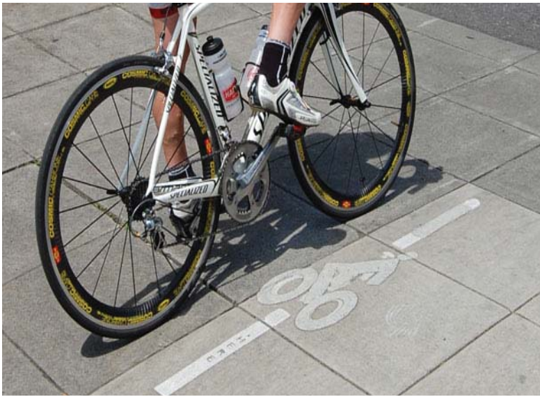
BICYCLE LOOP DETECTOR Enables cyclists to trigger signals at lights without needing to dismount. Photo credit: NACTO
