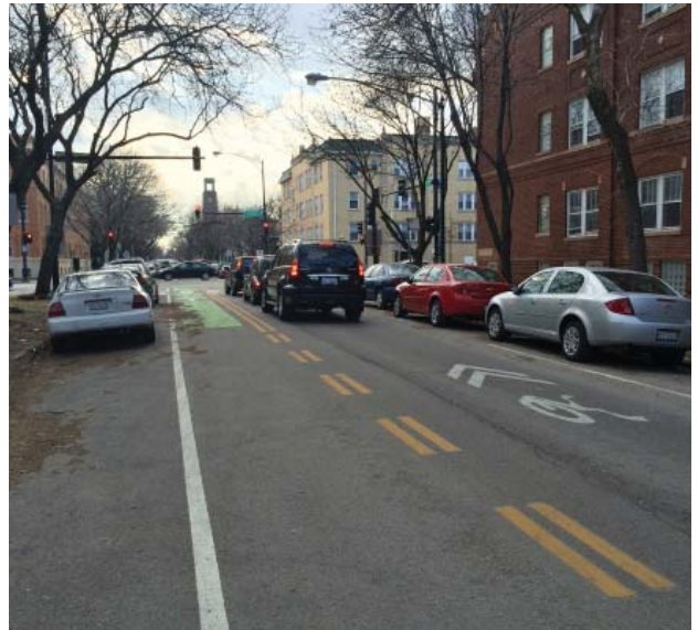
DASHED YELLOW LINES Help drivers and cyclists understand the appropriate lane position.
