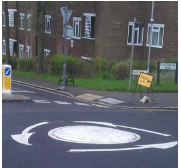
PAINTED MINI ROUNDABOUTS May be used prior to permanent installation, though they are not as effective. Photo credit: http://www.lbc.co.uk/
