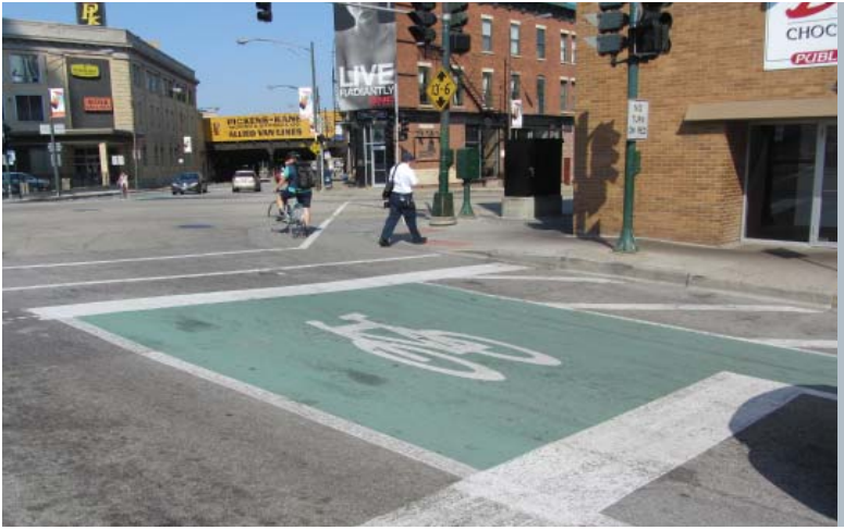
BIKE BOX Use at signalized intersections and place between the crosswalk and stop bar.
