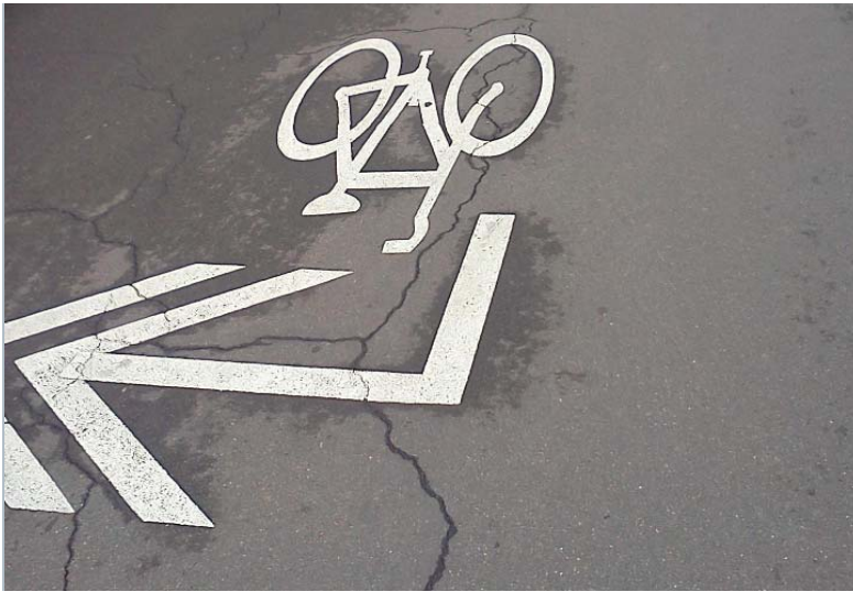
NEIGHBORHOOD GREENWAYS PAVEMENT MARKINGS WITH TURN ARROW Are used where Greenways are offset, jog, or where two Greenways intersect. Photo credit: J. Maus
