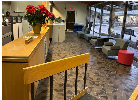
Hexagonal clay tile throughout interior and exterior of Village Hall.
