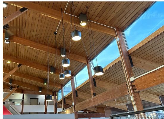
Bands of clerestory windows throughout interior of Village Hall.
