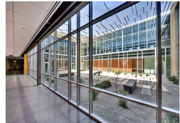
Curtain wall surround the interior courtyard at GSA Office Building (2019) in New Mexico, designed by Page Southerland Page
