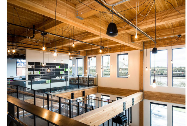
Exposed glulam timber structural beams at 38 Davis building (2016) in Portland, designed by Ankrom Moisan Architects
