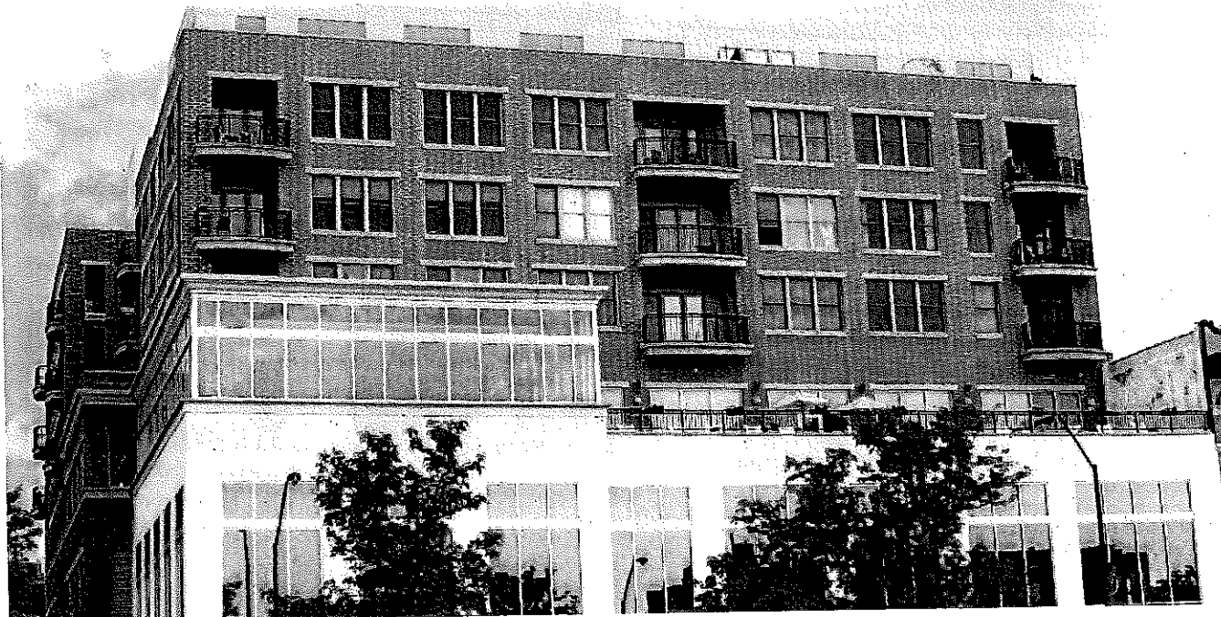
Another example of downtown mixed use buildings in Oak Park.
