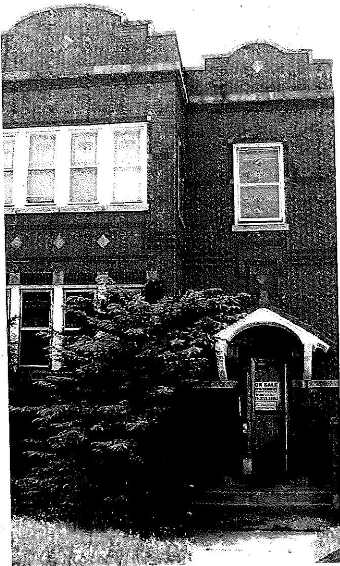
Foreclosure filings have increased especially in small multifamily buildings.
