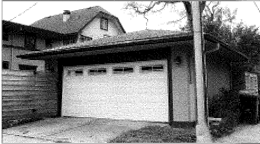
View of the garage which faces Thomas Street.
