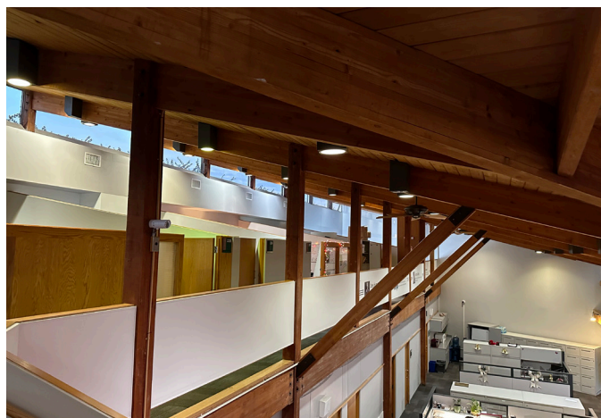
Exposed wood structure, ribbon windows below roof, and pony walls dividing offices at Mezzanine
