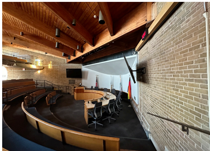
Council Chambers; brick cladding, exposed wood structure, semi-circular seating, exposed concrete balcony with metal bar railings
