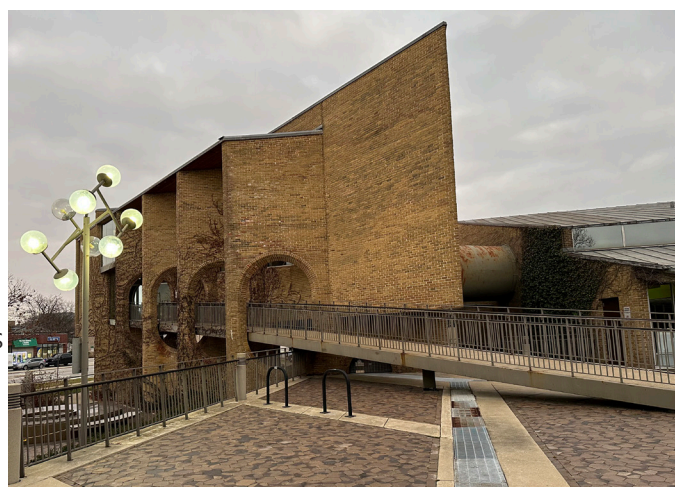
Common brick cladding, hexagonal clay tile pavers and globe light fixture at courtyard, and ramp through pylons leading to the Council Chambers
