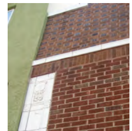
Build up of stucco material compared to neighboring building
