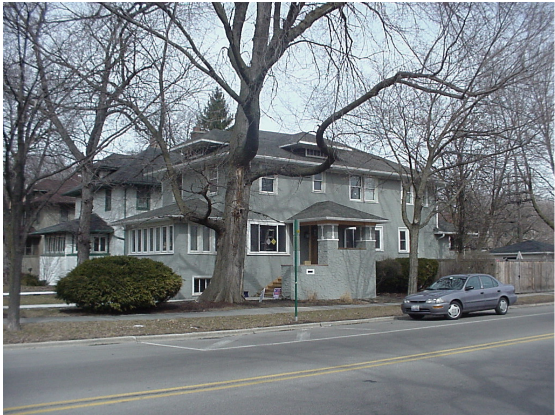
500 N. Elmwood Avenue (REHABILITATION) Gil Davies House, George Pearson, 1922 Trenis Jackson and Helen Thornton (owners) Patrick Loughran (architect) Goran Jelac, Wood Excellence (contractor)
