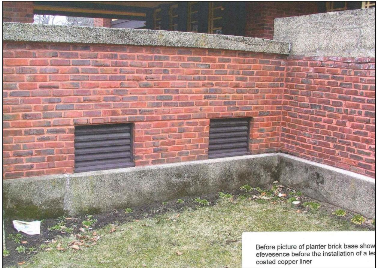
Before picture of planter brick base showing efflorescence before the installation of a lead coated copper liner
