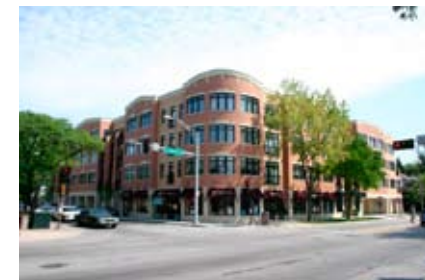
Figure 5.11: Twenty-first century development in the corridor has included multi-unit residential and mixed use buildings such as this recently completed four-story building at Ridgeland Avenue and South Boulevard.
