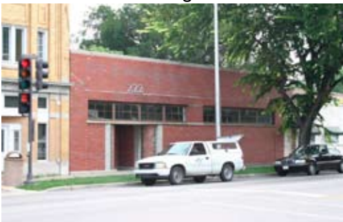
Figure 5.19: Non-contributing buildings include mainly post-World War II buildings like 222 Lake Street
