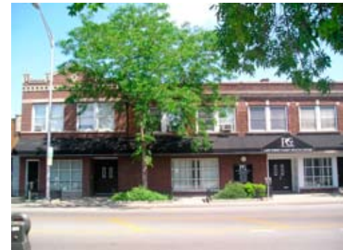
Figure 6.04: PCC Community Wellness Center on Lake Street
