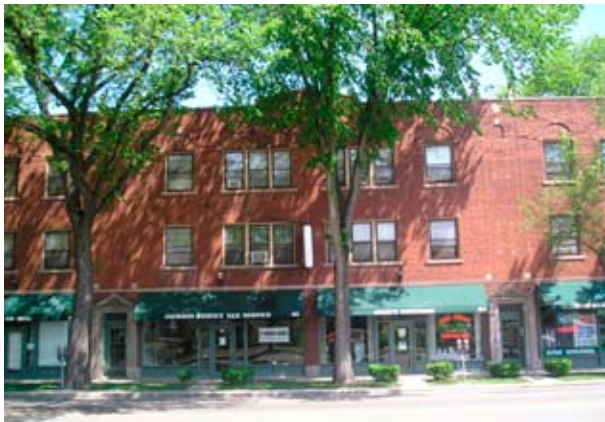
Figure 7.05: Mixed Use Building at the corner of Humphrey
