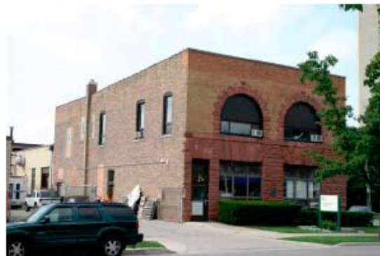
Figure 5.05: The building today, which now houses the Oak Park main water pumping station.
