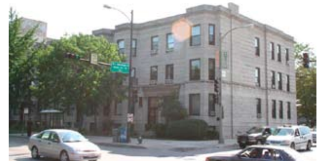
Figure 7.09: Multi-family building on Austin Blvd.
