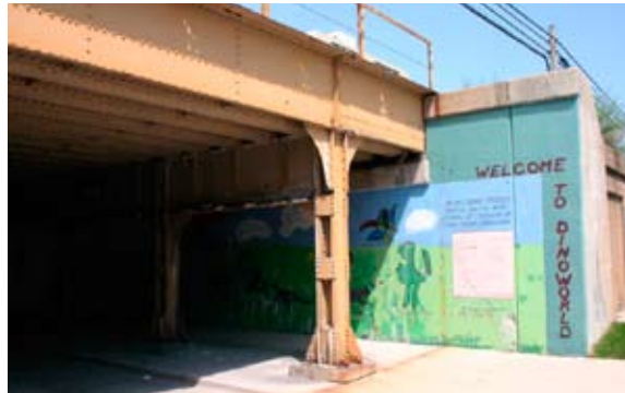
Figure 1.08: CTA Viaduct Underpass
