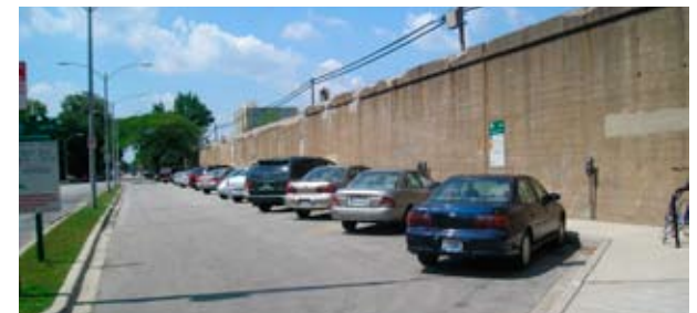
Figure 1.09: Parking Along Viaduct
