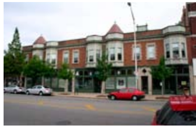
Figure 5.21: Part of the commercial strip on Lake Street near Ridgeland Avenue.
