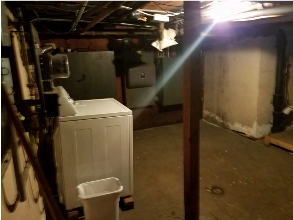
The interior of the basement.
