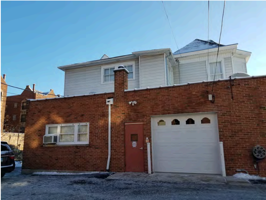
The exterior southwest side of the Site.
