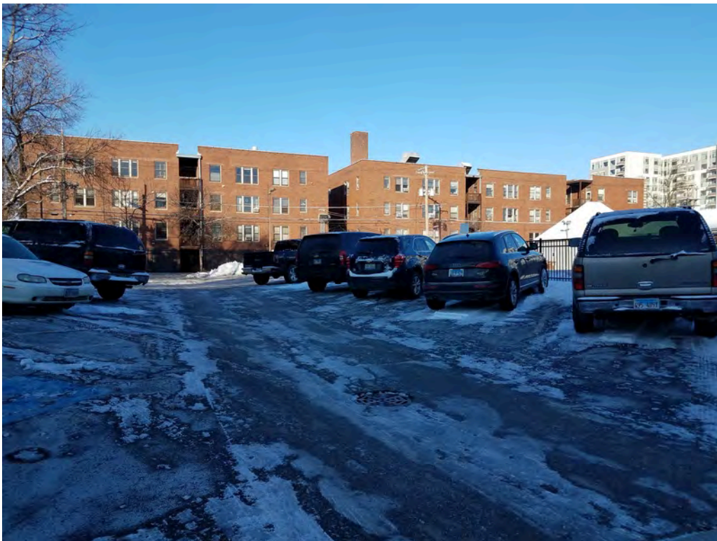
The adjoining properties to the south.
