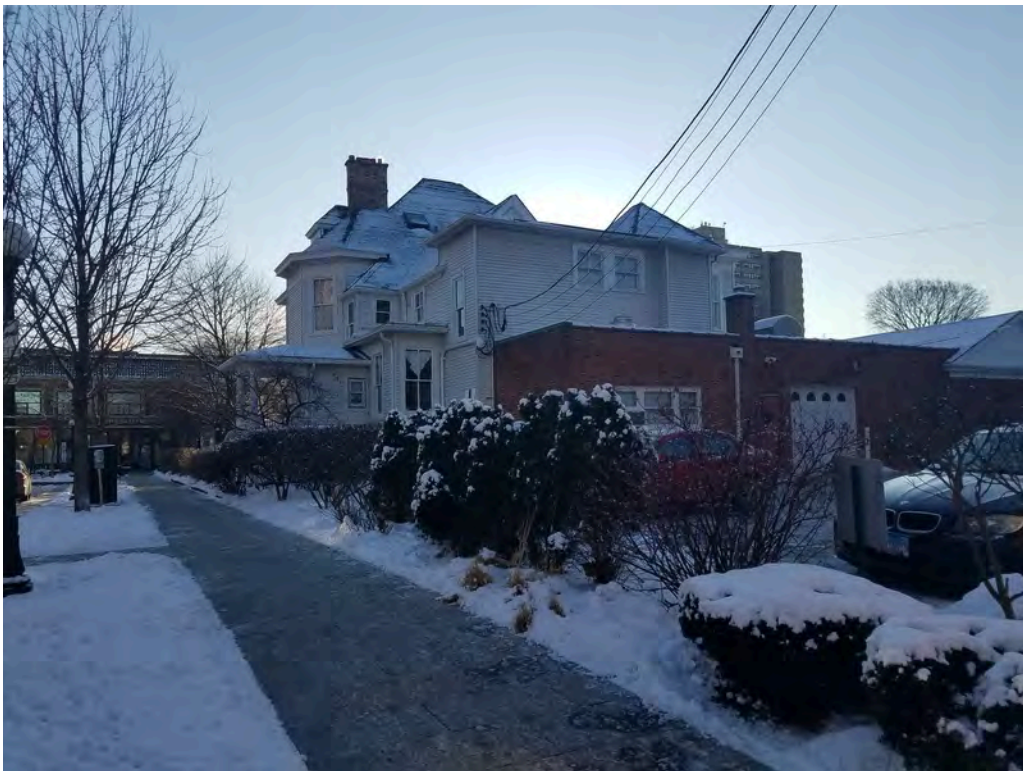
The exterior north side of the Site.
