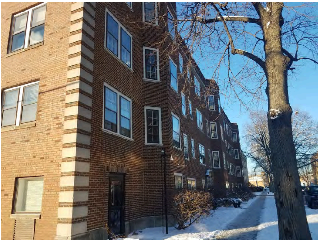
The adjoining properties to the west.
