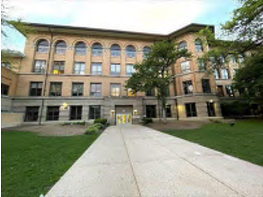
North End of OPRF Scoville Facade - 4 Stories
