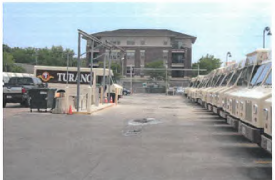
Right: Pump Island - Out of Service Gasoline UST
