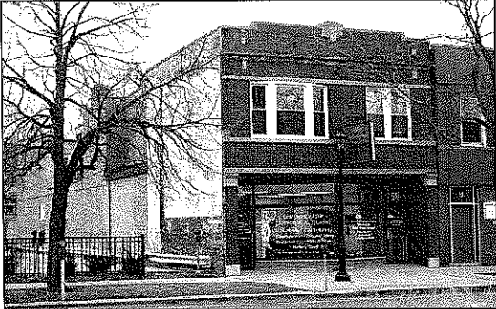
58 Madison Street (1921) (Source: Cook County Assessor)
