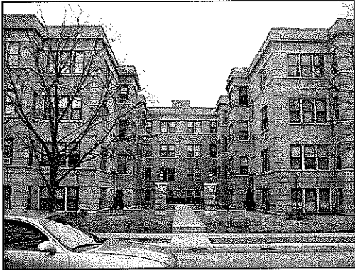
1158-64 S. Oak Park Avenue (1924) (Source: Village of Oak Park)
