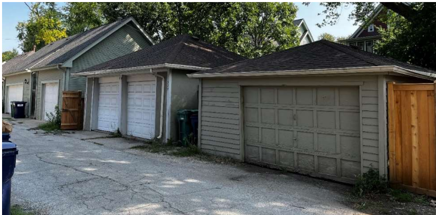
Alternate view from alley, south garage on the right and north garage on the left.
