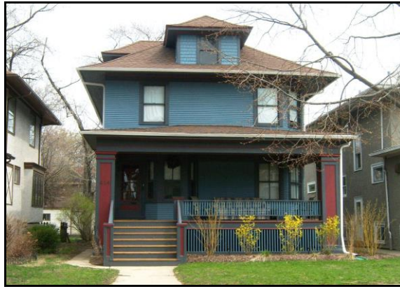
814 Clinton was destroyed by fire
