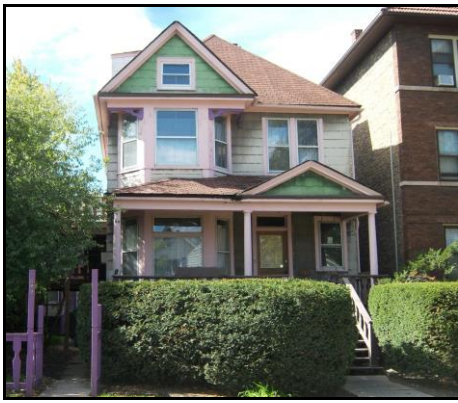
541 N. Humphrey was destroyed by fire
