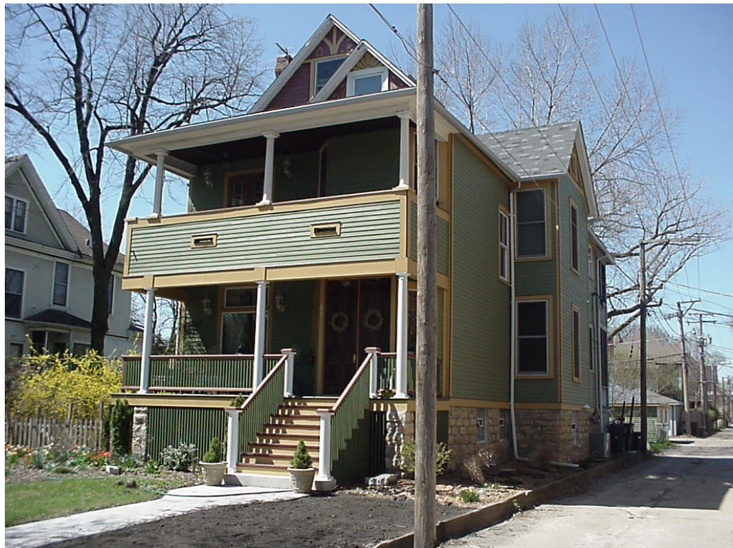
115 Wesley Avenue (RESTORATION) Beth Sievert Pat Magner, Architect
