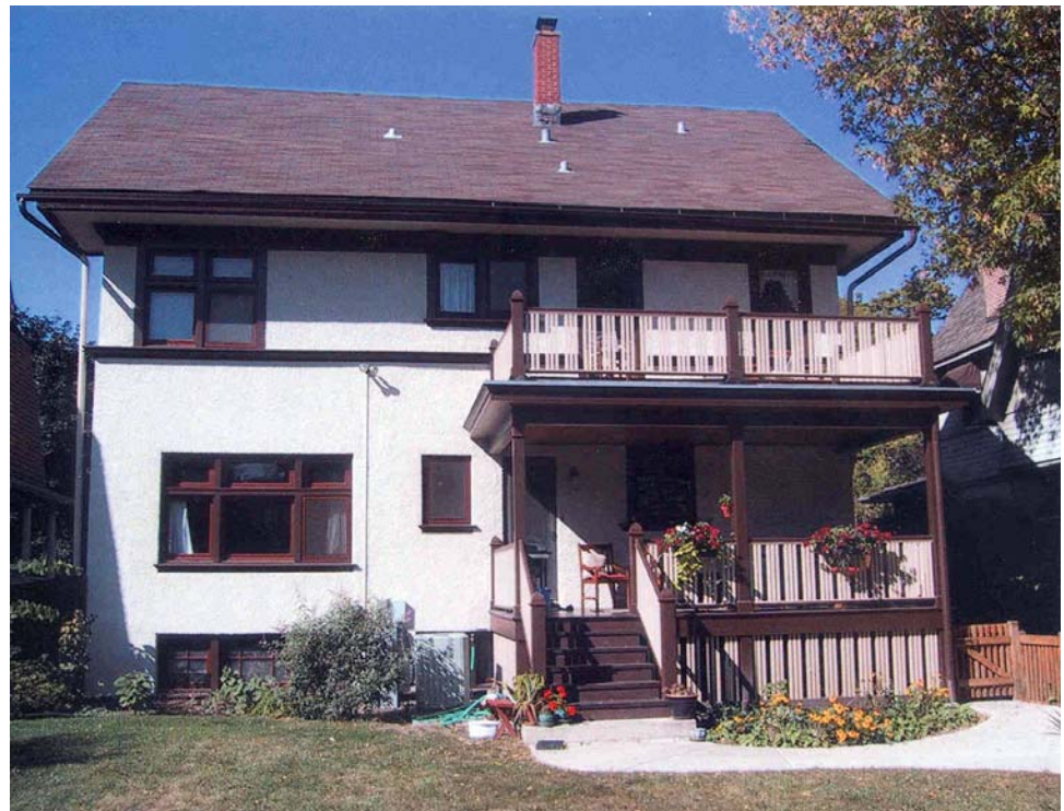
410 N. Elmwood Avenue (RESTORATION OF REAR PORCH) F. W. Pringle House, 1908 Donald and Bonnie Chauncey Von Dreele-Freerksen Construction Co.
