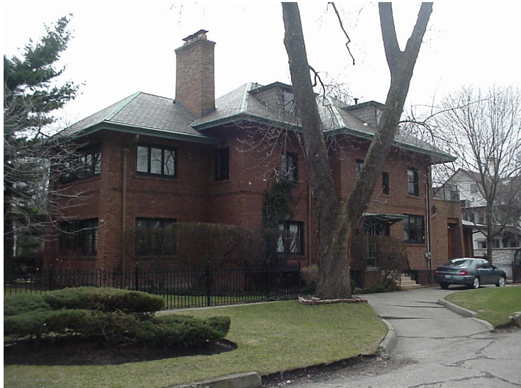
701 Columbian Avenue (RESTORATION, SIDE ADDITION) Curtis Camp House, Charles E. White, 1915 Terry and Jana McIlroy Anthony Ronning, Architect Von Dreele-Freerksen Construction Co.
