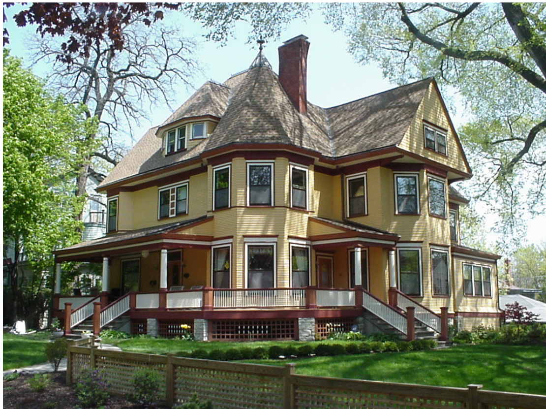
320 N. Euclid Avenue (RESTORATION) Steve and Julie Scheuring A.C. Remodeling
