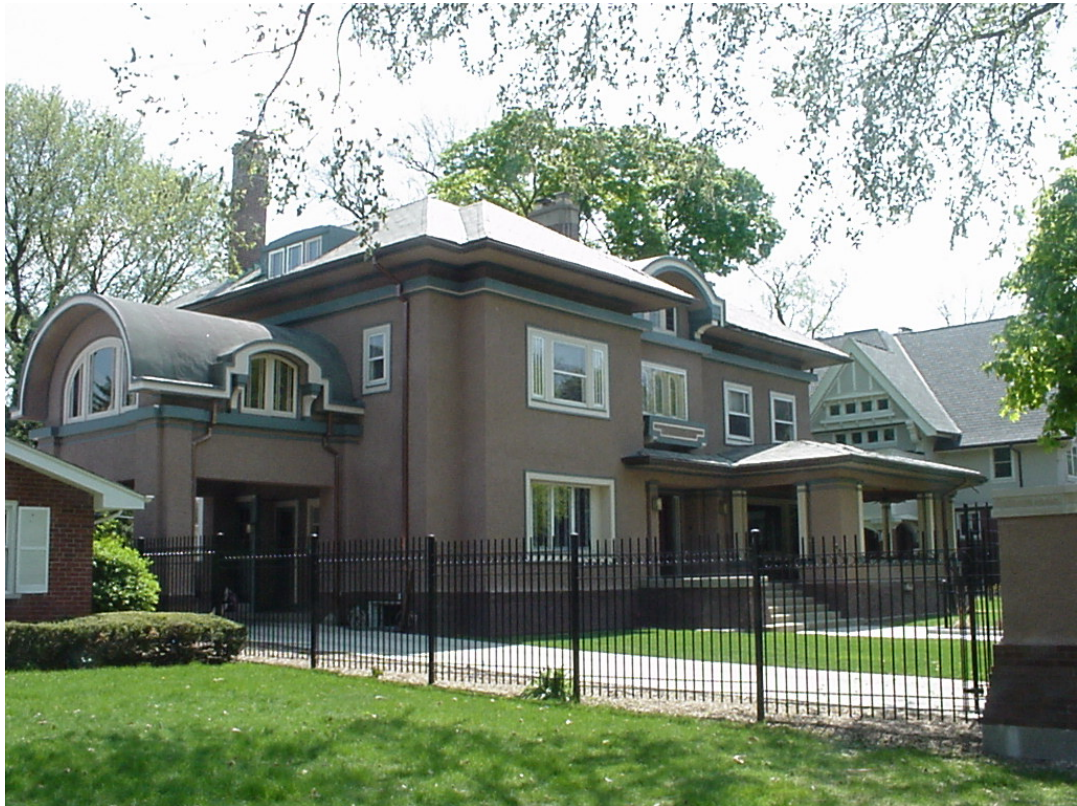
630 N. Euclid Avenue (RESTORATION OF EXTERIOR) L. V. Dougherty House, George Maher, 1906 Susan Price and Marc Martinez Von Dreele-Freerksen Construction Co.
