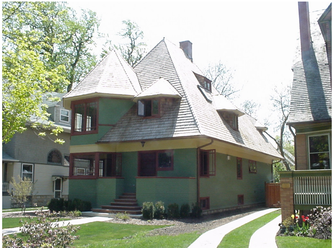
1027 Chicago Avenue (RESTORATION, REAR ADDITION) Thomas Gale House, Frank Lloyd Wright, 1893 Jim Dee and Brent Kaufman DMA Architects/Northstar Studios The Heartland Construction Group
