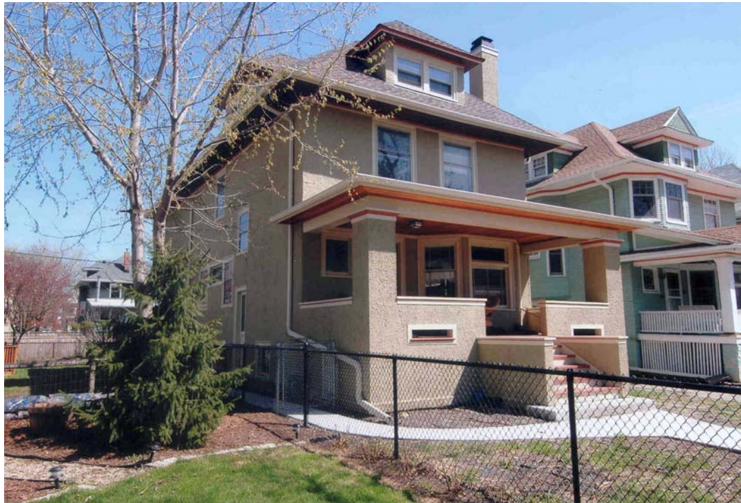
732 Gunderson Avenue (RESTORATION, REAR ADDITION) S. T. Gunderson & Sons, 1909 Miles and Susan Harris Lineworks Ltd., Architect Von Dreele-Freerksen Construction Co.
