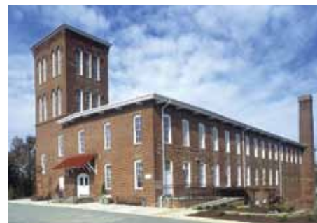
Prizery/R.J. Reynolds Tobacco Warehouse, South Boston, Virginia (1900). Rehabilitated for commercial use. Photographs: Ian Bradshaw.
