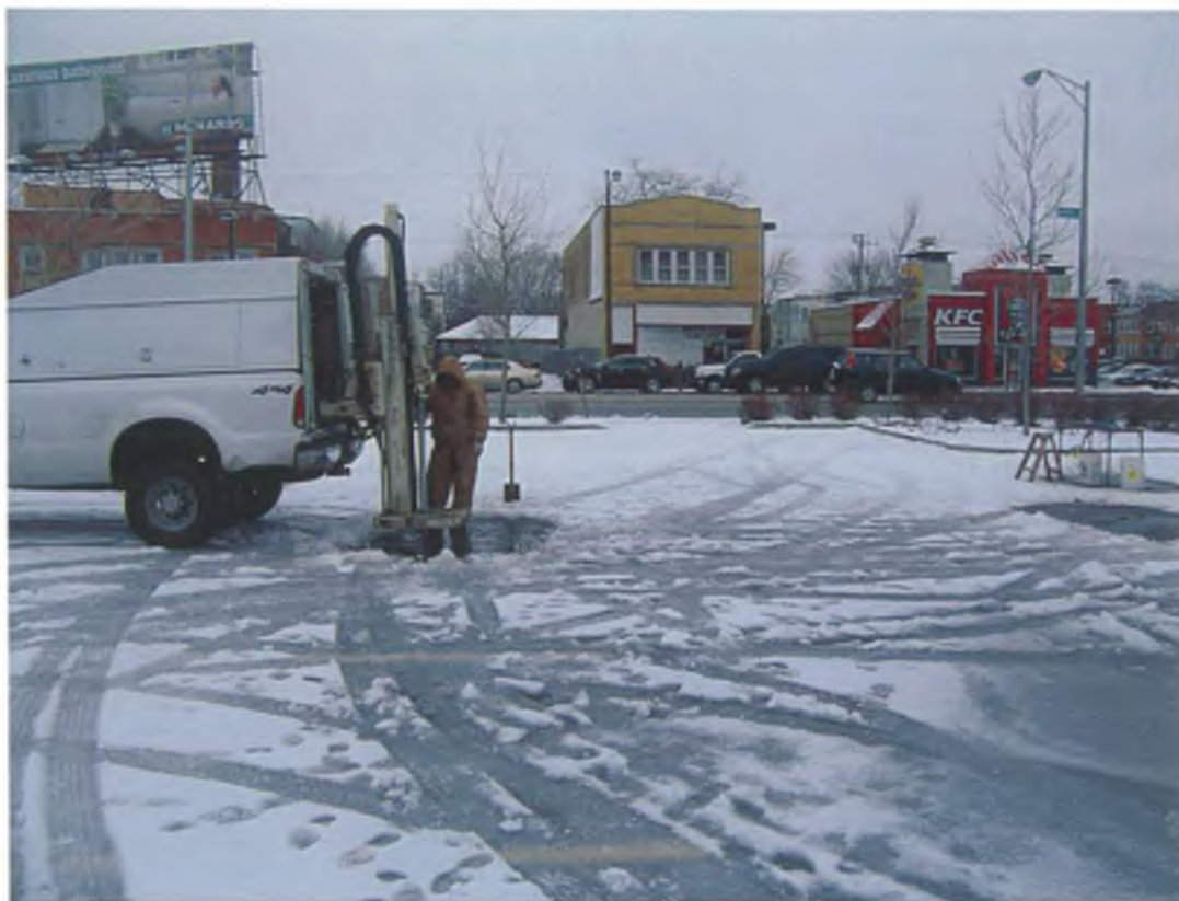
Boring B4, viewed from South (Boring B1 to far right)
