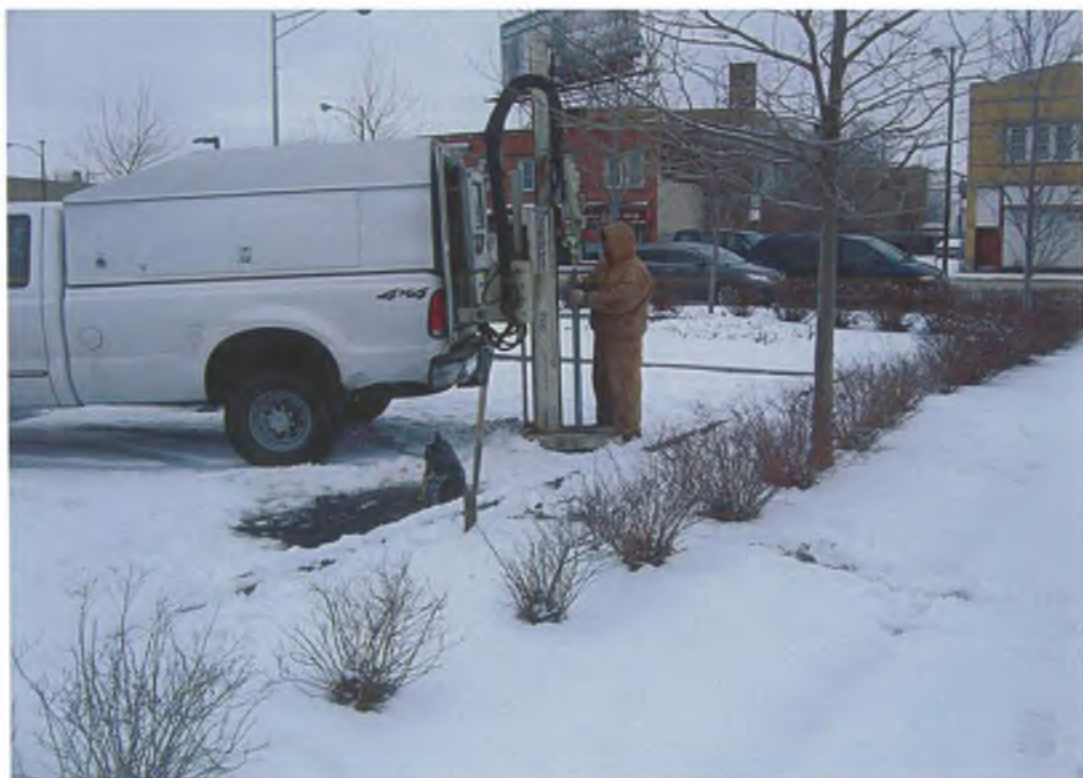
Boring B3, View from Southeast (Refusal Boring to Left)
