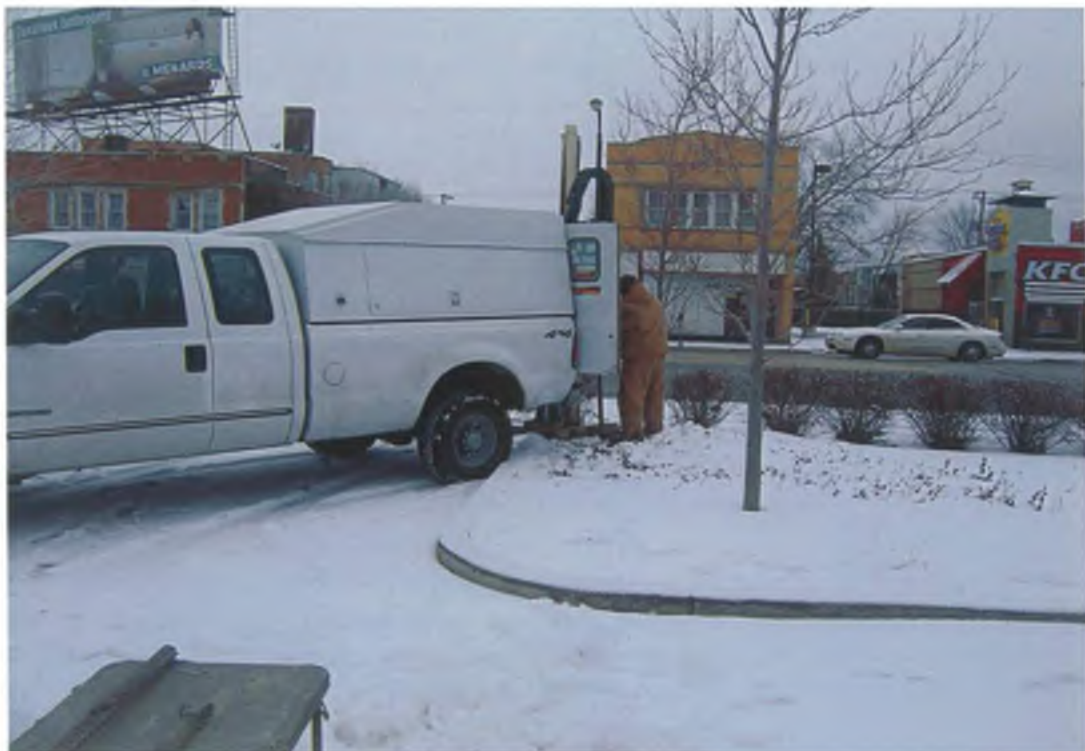
Boring B2, View from South
