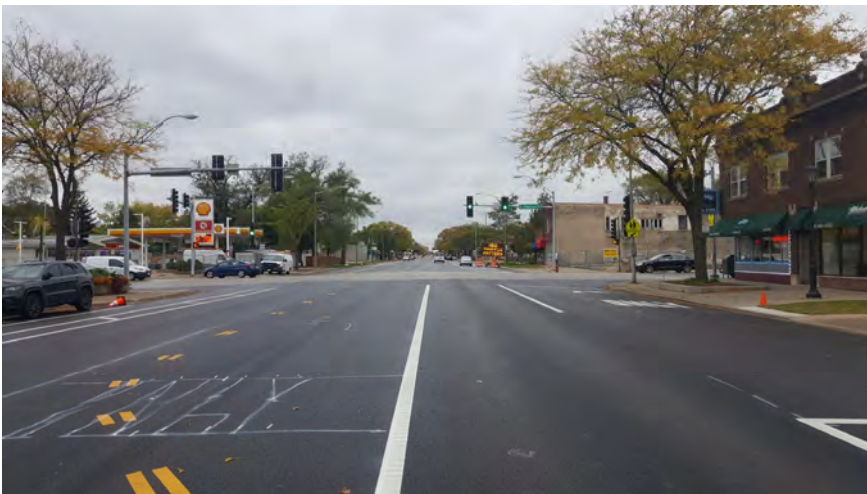
Westbound Madison St (Ridgeland Ave intersection)
