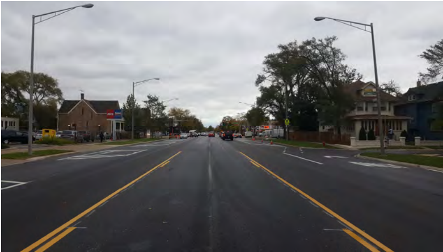
Eastbound Madison St (Elmwood Ave intersection)
