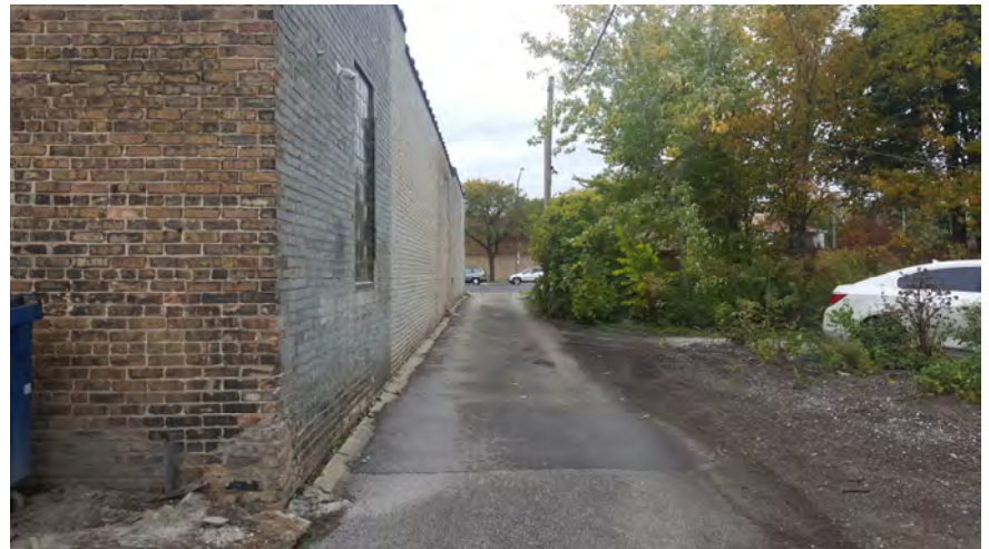
Northbound Public Alley (South of Madison St, East of Site)
