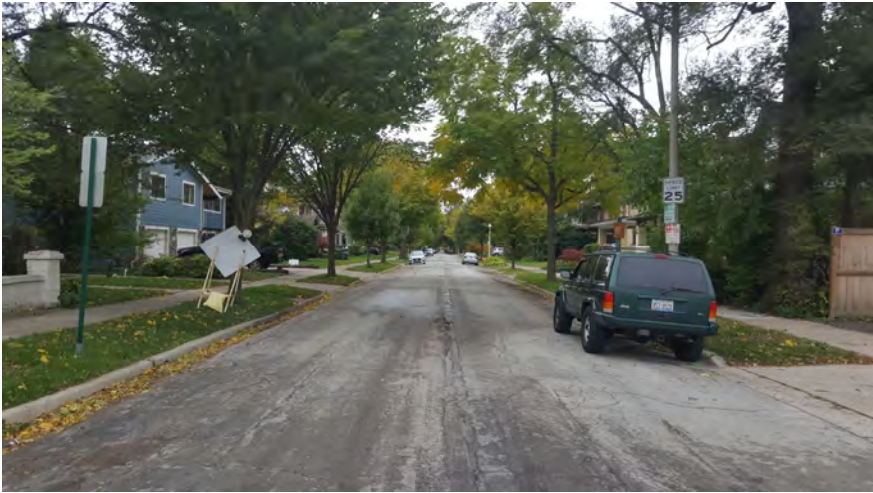
Southbound Elmwood Ave (South of Madison St)
