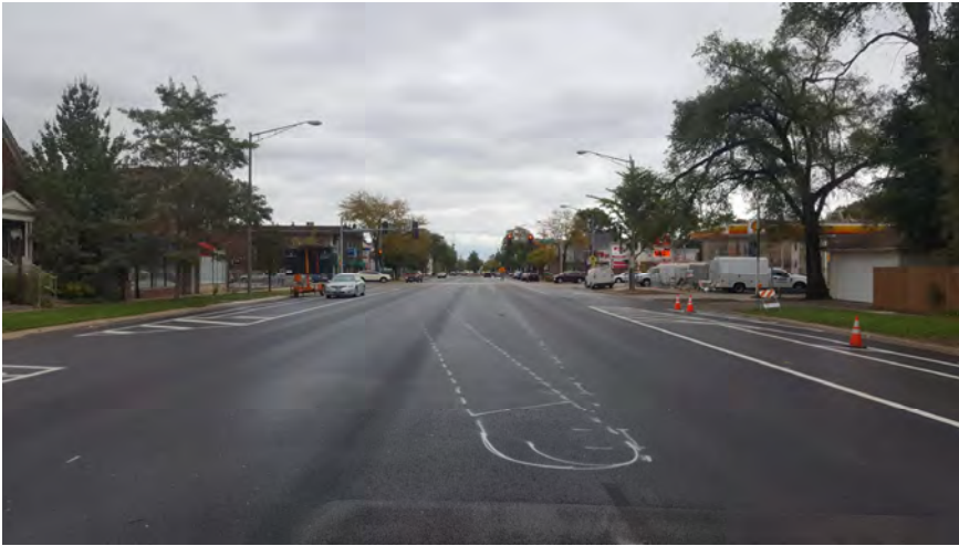
Eastbound Madison St (Ridgeland Ave intersection)
