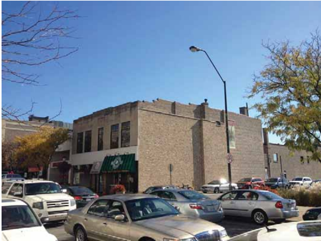
05-NORTH BUILDING SITE - VIEW TO SOUTHEAST
