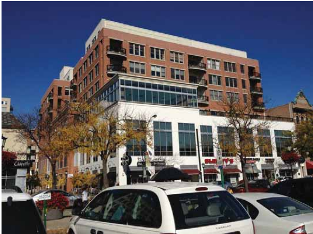
12-MAPLE AVENUE - VIEW OF LAKE STREET
