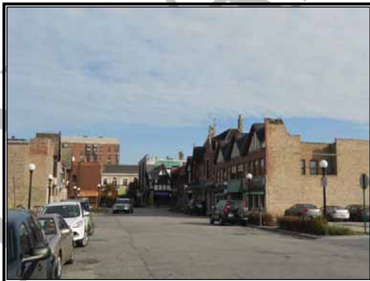
View east from the subject site
