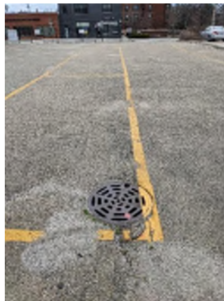
South end of property, storm drain, facing North
