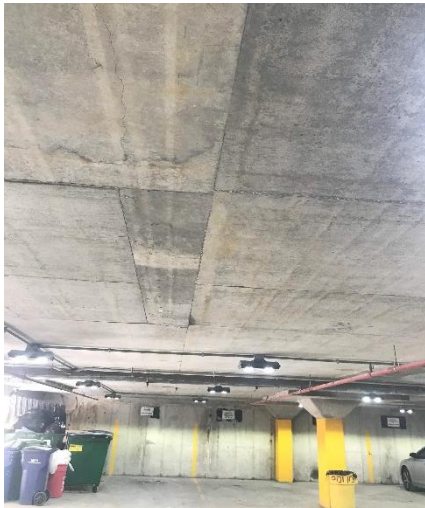
Repaired concrete deck at garage
