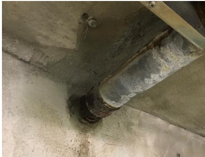
Repaired conduit within garage
