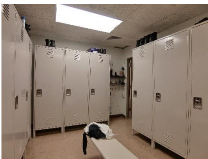
Lack of storage within sergeant's locker room
