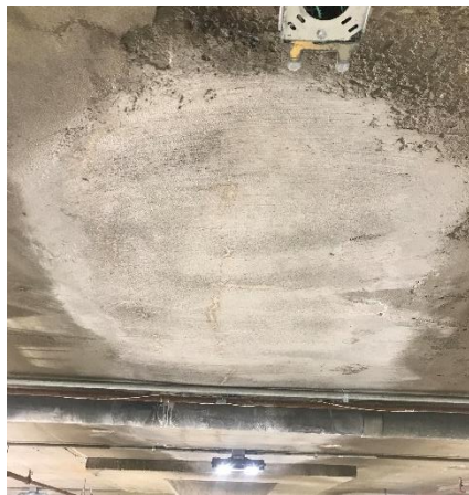
Area of patched concrete deck at garage
