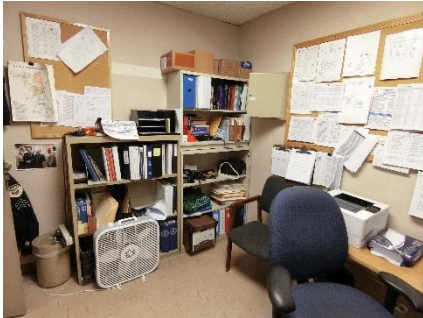
Supplemental fans located throughout building to help circulate air
