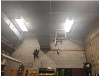
Existing back of house lighting fixtures
