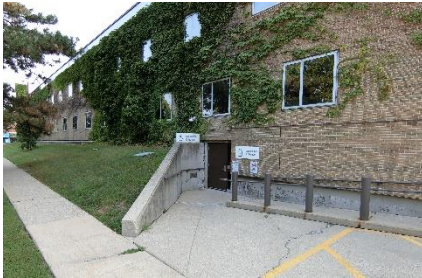
Lack of wayfinding to ADA ramp
