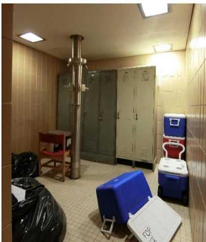
Men's shower being used for storage
