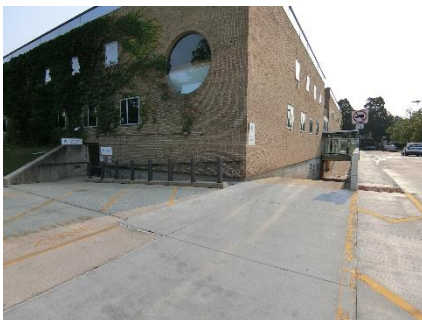
View looking North East
