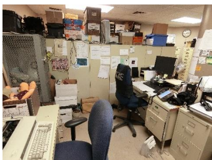
Boxes being stored too close to the ceiling
