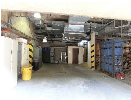
Unsecured access from Sally port to building storage
