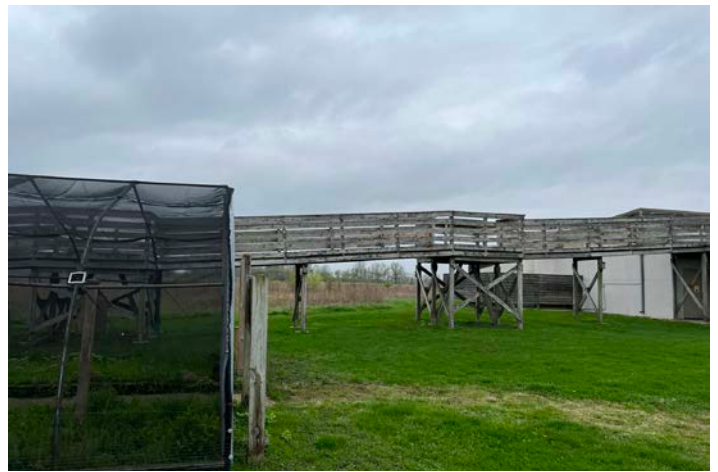
Exterior Conditions from Assessment Site Visit
