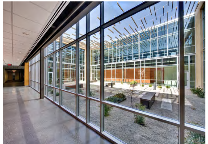
Curtain wall surround the interior courtyard at GSA Office Building (2019) in New Mexico, designed by Page Southerland Page
