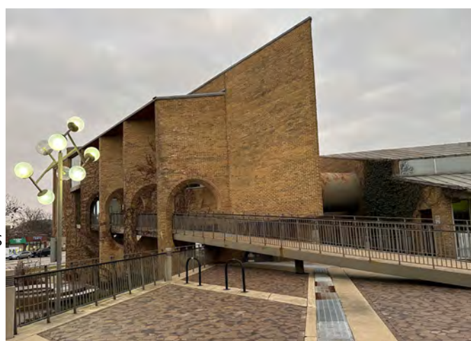
Common brick cladding, hexagonal clay tile pavers and globe light fixture at courtyard, and ramp through pylons leading to the Council Chambers
