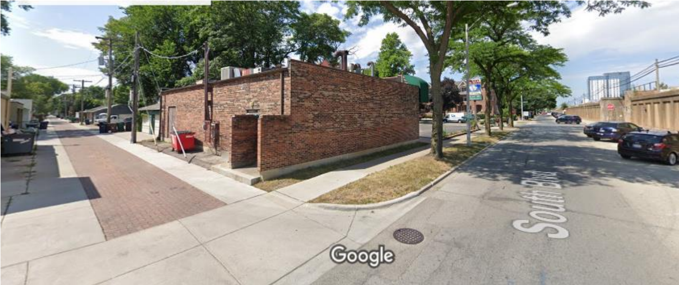
VIEW FROM PUBLIC ALLEY & SOUTH BLVD.
