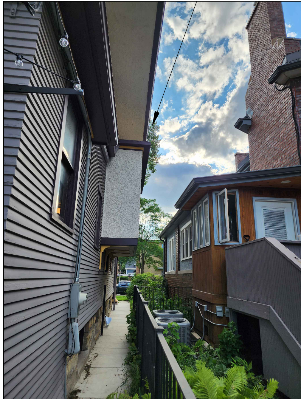
LOOKING NORTH WEST
