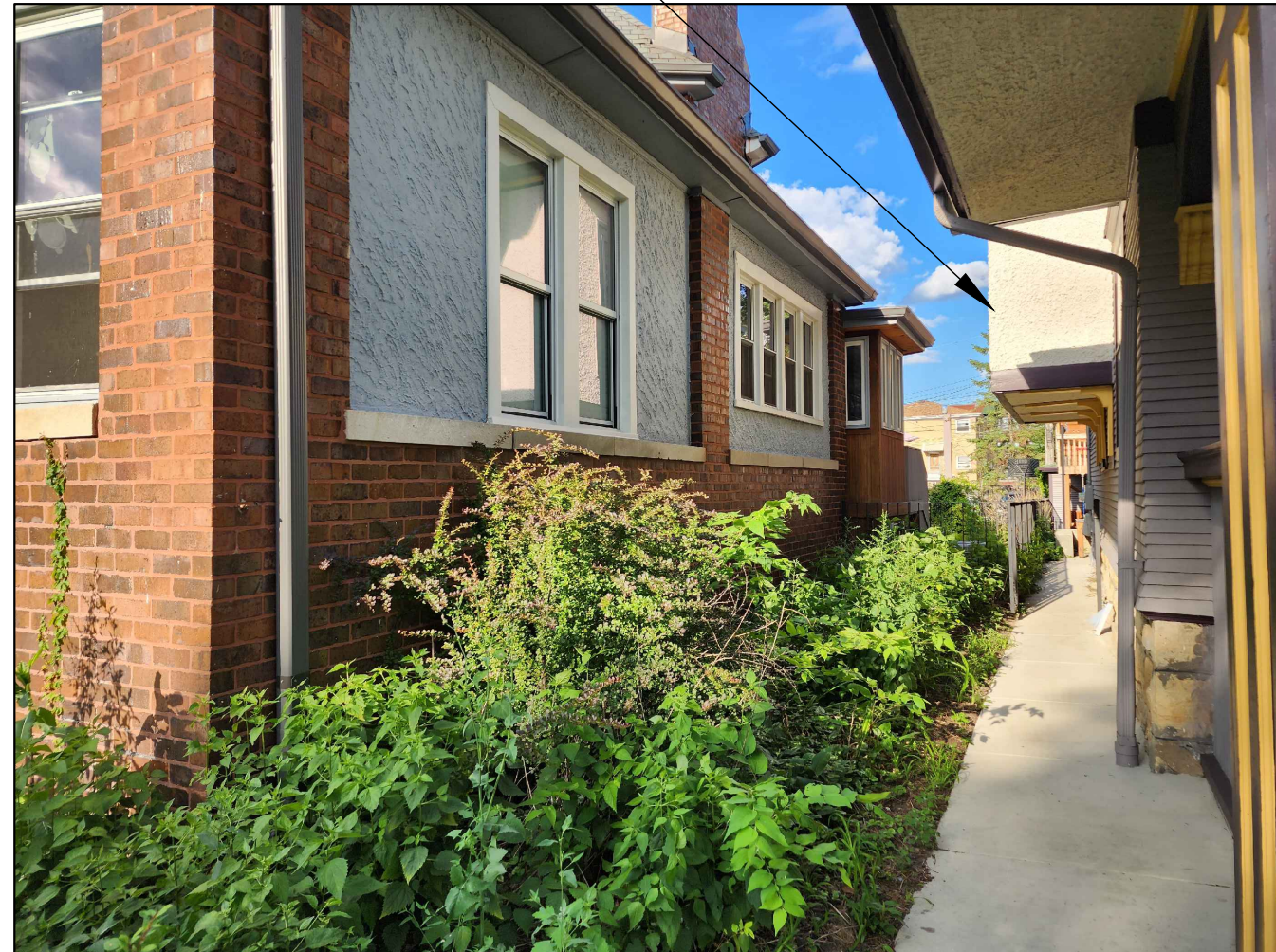
LOOKING NORTH EAST
