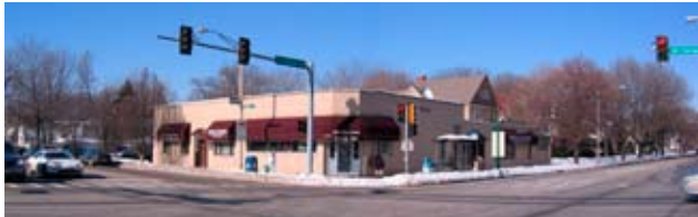
Figure 6.05: North West corner of Ridgeland Intersection
