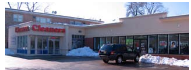
Figure 5.04: Parking Lot at Chicago - Ridgeland intersection
