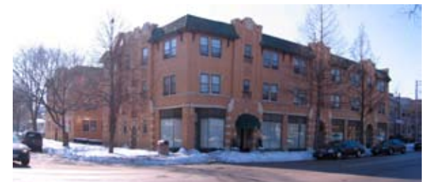
Figure 3.09: Multi-family residential building at the corner of Chicago & Humphrey.
