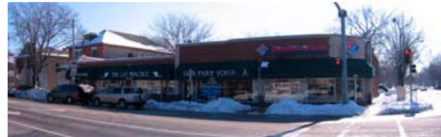
Figure 6.09: South East corner of Ridgeland Intersection
