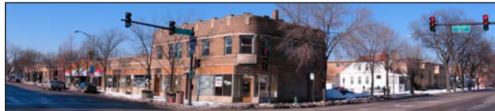
Figure 6.17: Austin Chicago Intersection -North -East Corner
