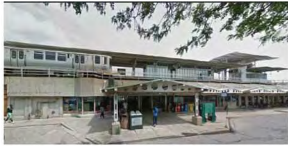
CTA Green Line Entrance at South Boulevard
