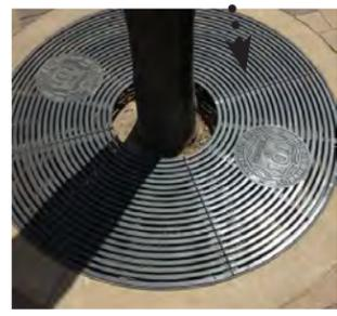
6' DIA. RAW DUCTILE IRON WITH KNOCKOUT RINGS
