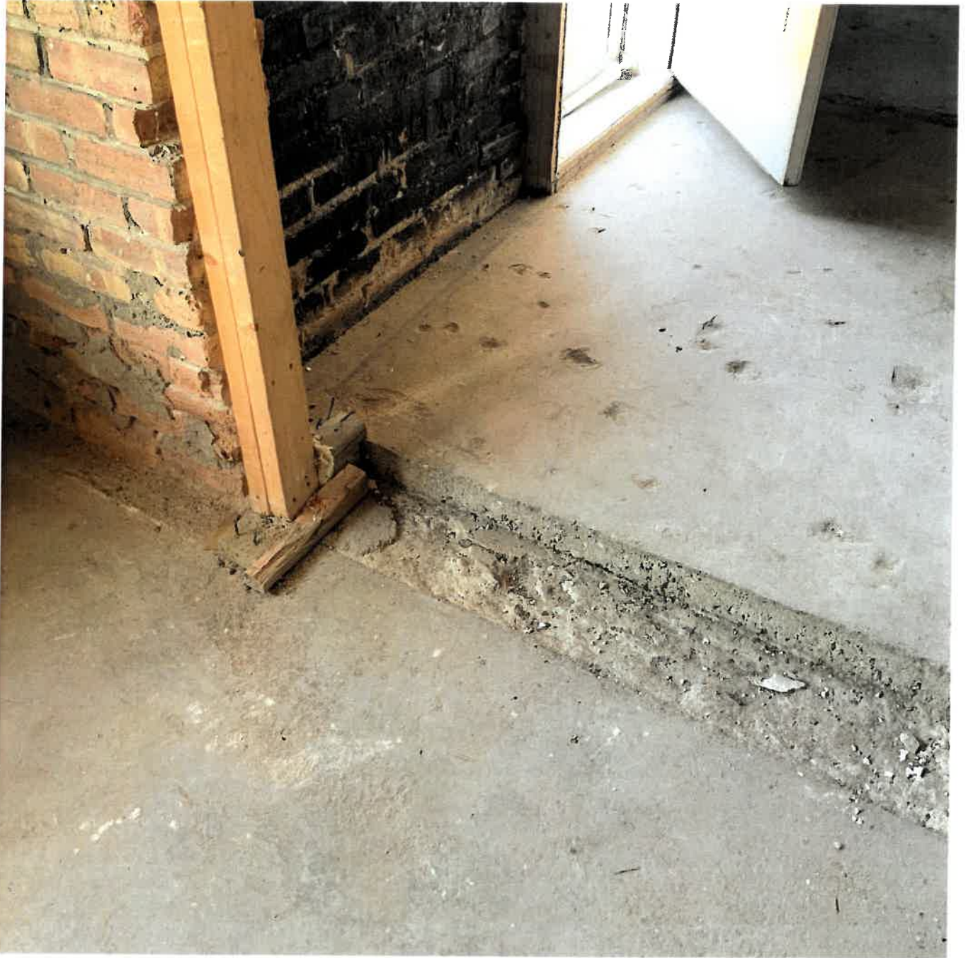
A three (3) inch depression exists as you enter the old garage bay.
