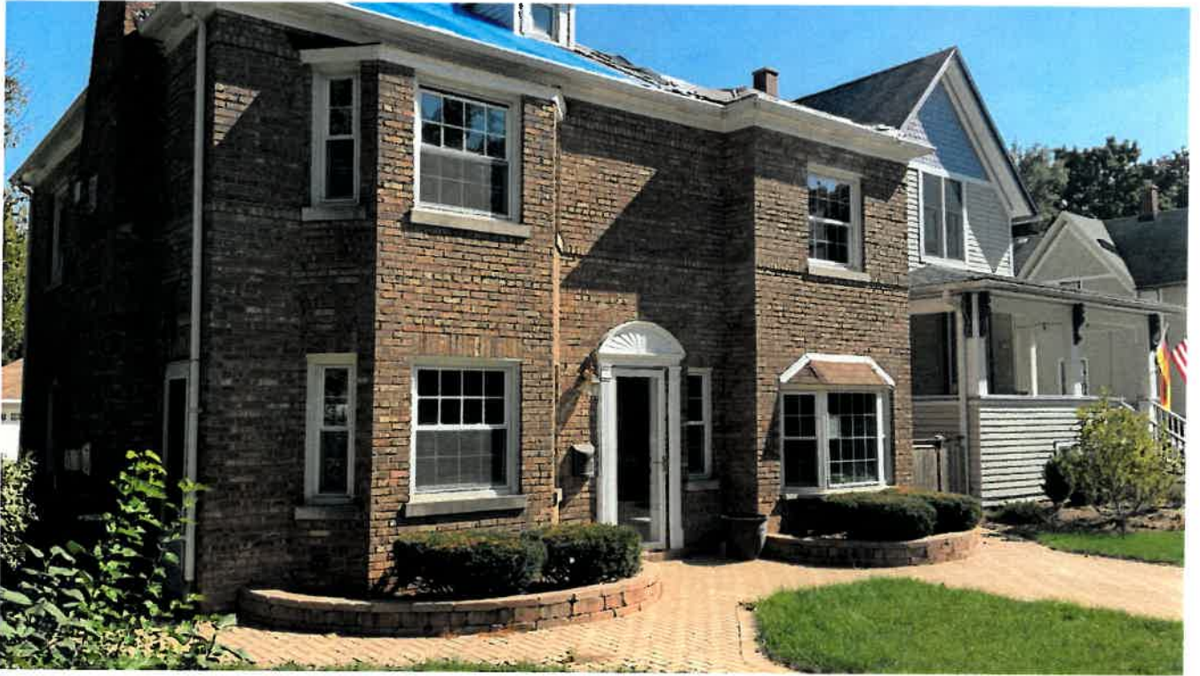
The Front Elevation with north side of the home.
