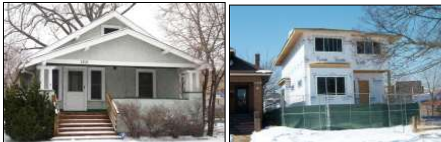
1231 Hayes was demolished in 2013, with the new house under construction
