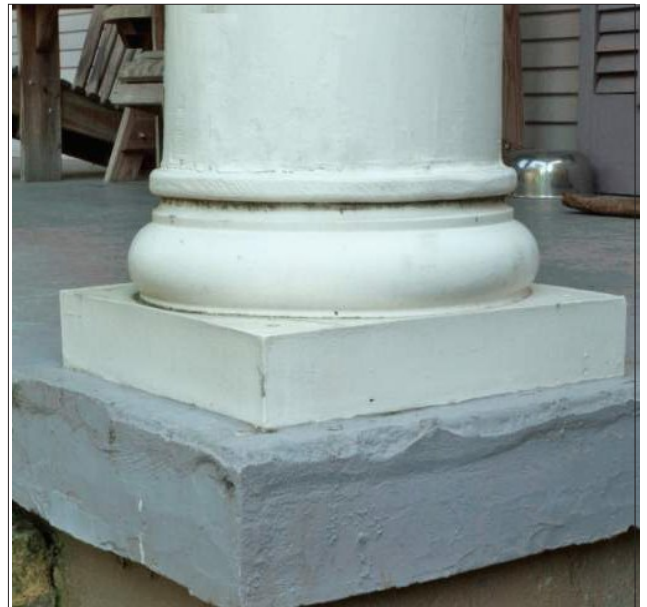
The porch column above is wood but the base has been replaced with a composite material that is visually similar to the former wood base.
