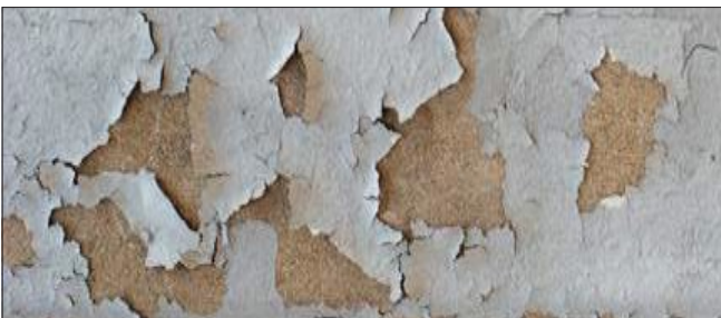
When painting stucco, it is recommended that breathable masonry paint be used and that loose or flaking paint be removed prior to repainting.
