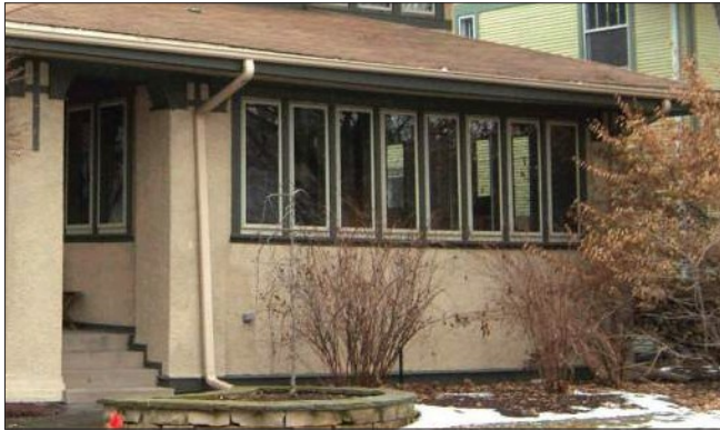
This porch has been partially enclosed with operable windows allowing the space to be used in the winter months.
