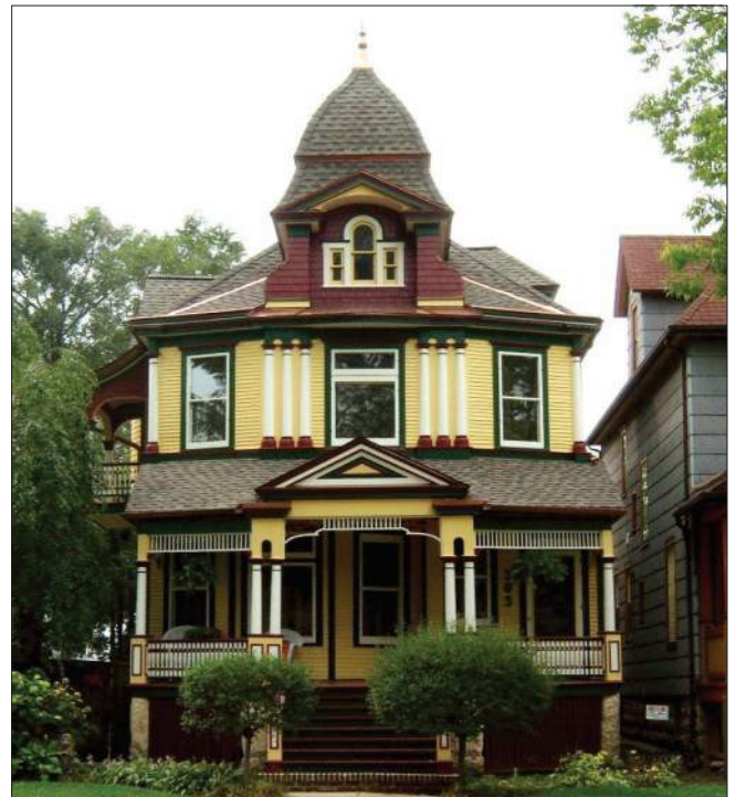
This house features a variety of exterior wood trim, ornament, and details that are highlighted by the paint scheme and would be difficult to replicate with artificial materials.
