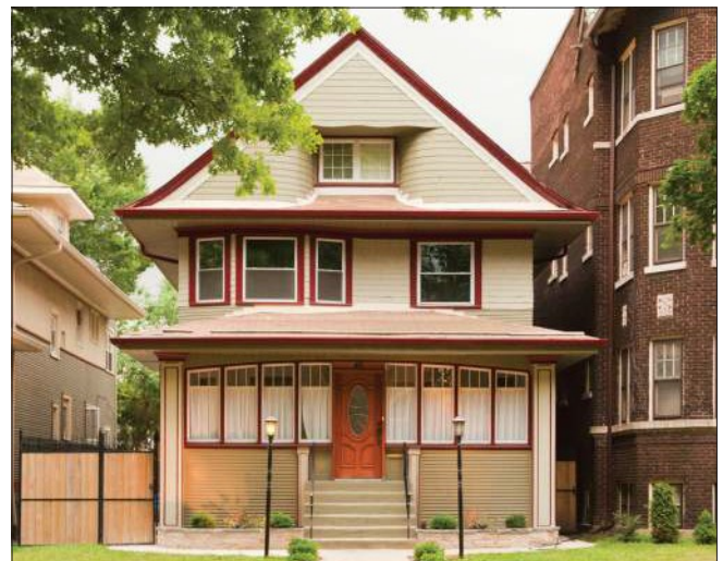
Enclosing a porch to provide more habitable space is an example of an alteration.
