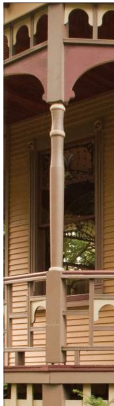
Turned Wood Post with Brackets
