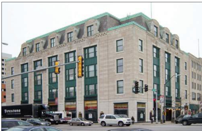
Many of the buildings in Downtown Oak Park, including this one, were constructed solely for commercial uses.
