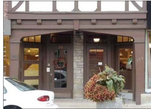
This alcove encompasses two storefront entrances and is capped by a Tudor Revival style cornice.
