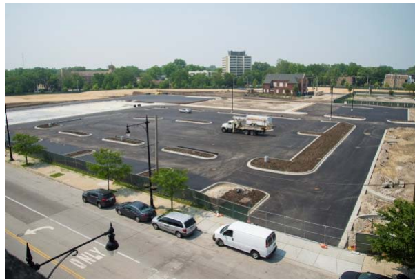
Completed Whole Foods Sitework
