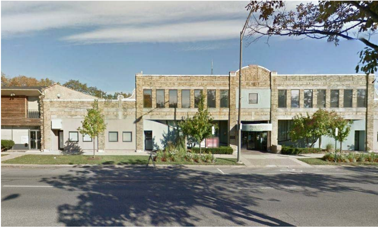
NORTH SIDE OF MADISON ST. ACROSS FROM SITE
