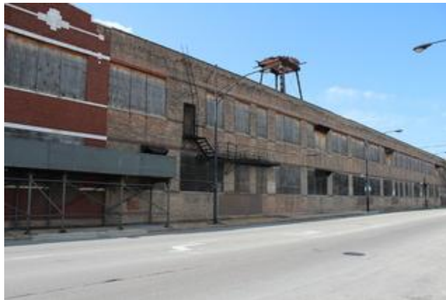
The shuttered Storkline Factory at 26th Street and Kostner Avenue. Mercy Housing Lakefront plans to turn the old factory building into multi-family rental units.
