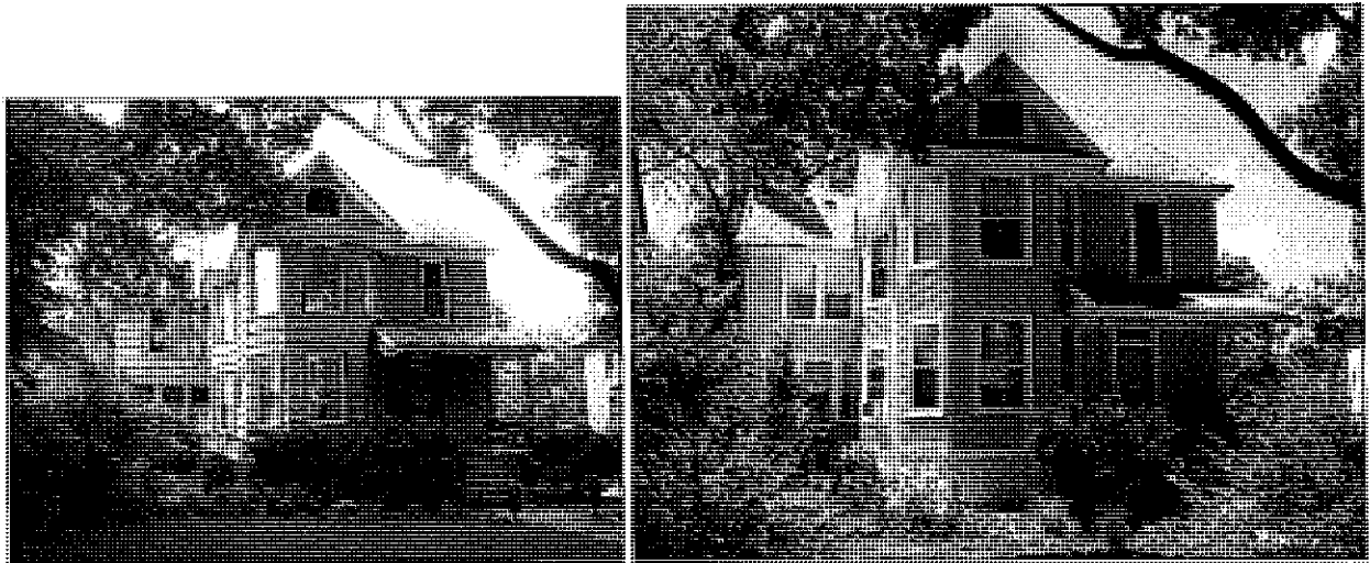
View of house before (L) and after (R) the removal of the asphalt siding
