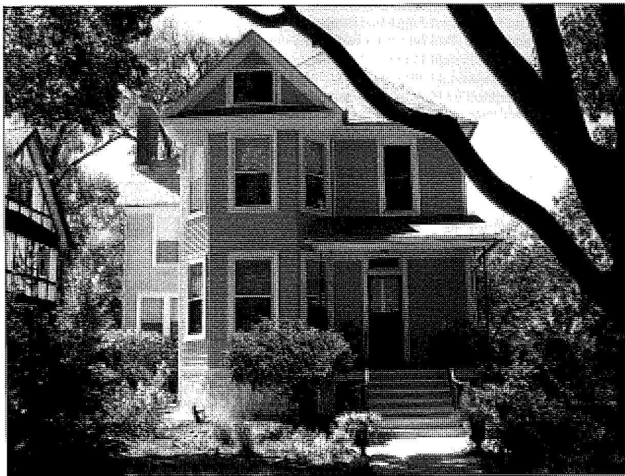
Rankin-Hemingway House 639 North Oak Park Avenue
