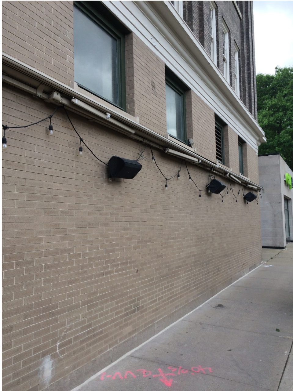
Photo 12: View of north elevation showing awning and speakers to be removed. Note the grill in the third window.
