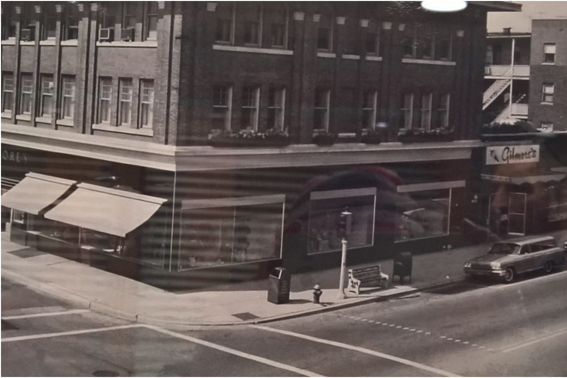
Photo 17: Circa 1950s view of the storefronts after the 1936 alterations of the storefronts. Note that the north elevation has large display windows and the corner entry has been eliminated.
