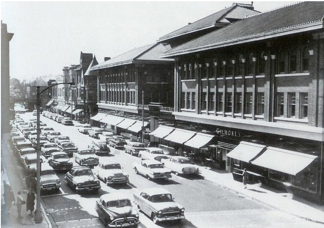
Photo 16: Circa 1950s view of the storefronts after the 1936 alterations. Note that all of the original storefront has been removed (the columns were retained and hidden behind the Vitrolite panels).
