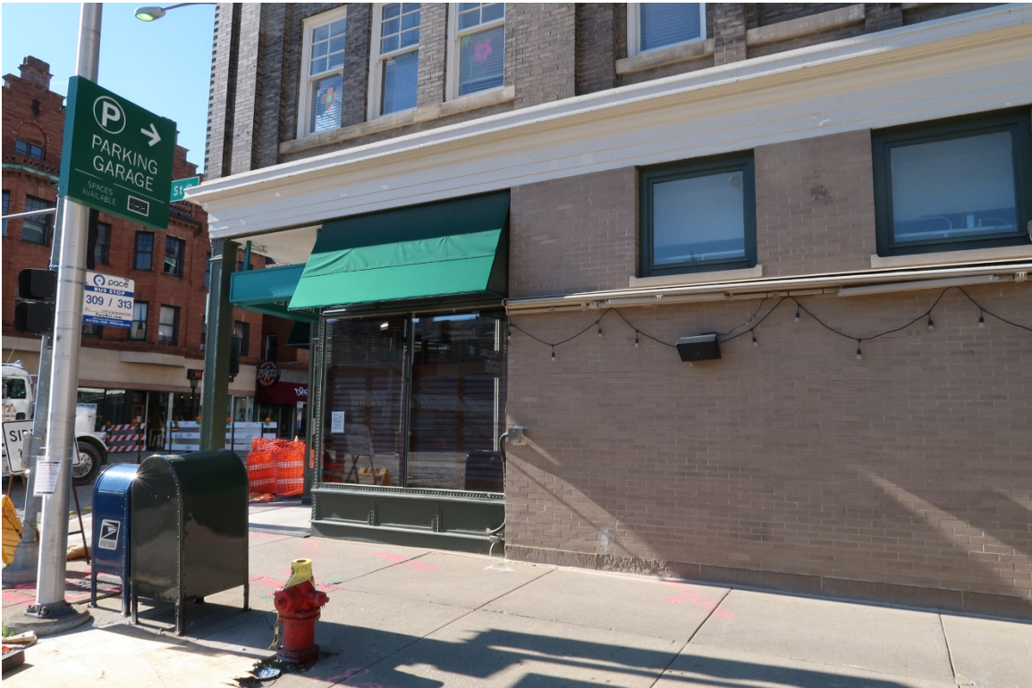
Photo 11: North elevation showing one bay of storefront, brick wall and clerestory windows.
