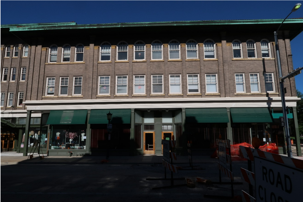
Photo 3: East elevation of storefronts.
