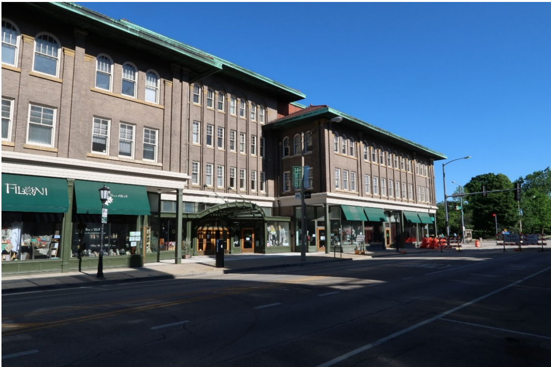
Photo 2: Scoville Square Building as seen from the south along Oak Park Avenue.
