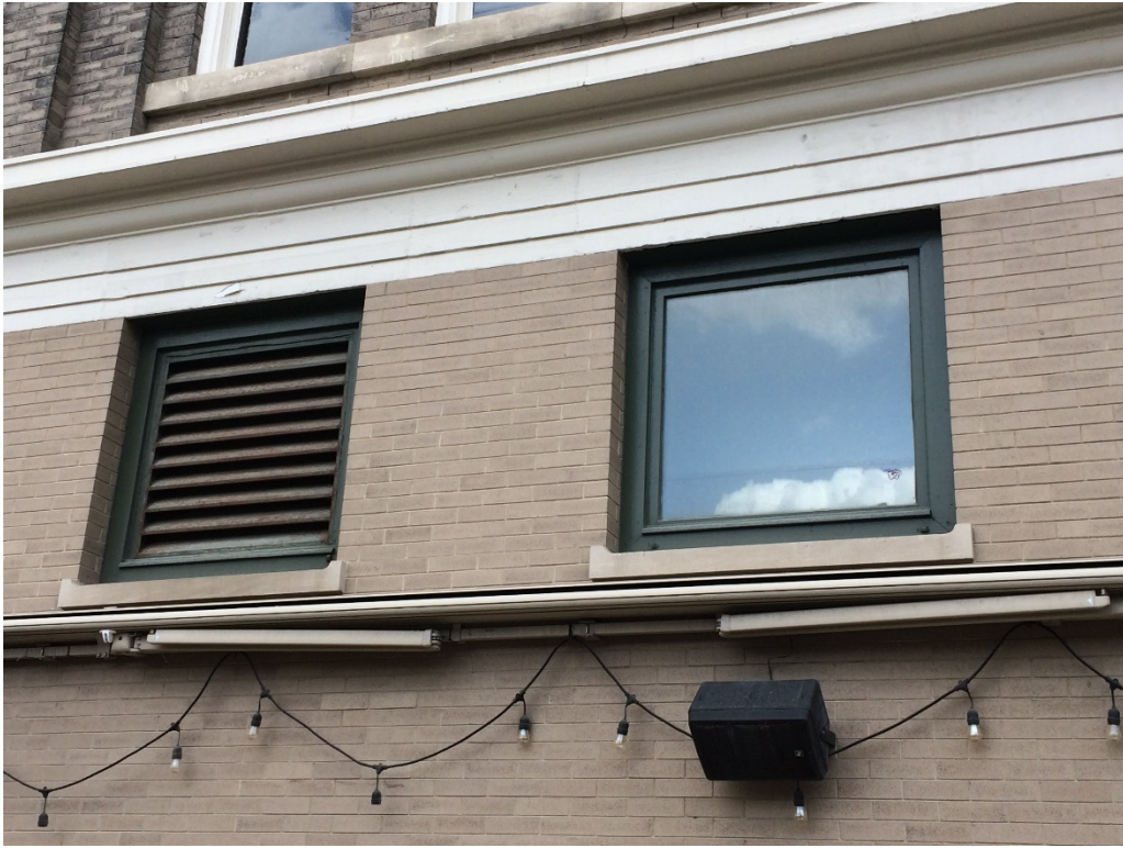
Photo 13: Detail of existing clerestory windows, one with a grill.
