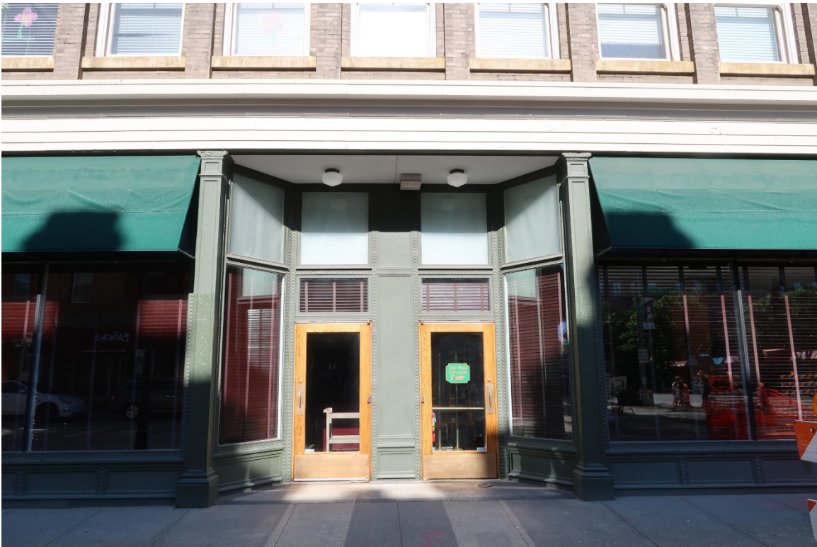
Photo 4: East elevation existing recessed entry.
