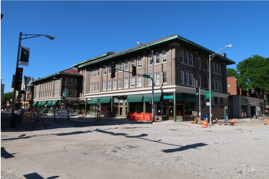
Photo 1: Scoville Square Building as seen from the northeast corner of Oak Park Ave. and Lake St.
