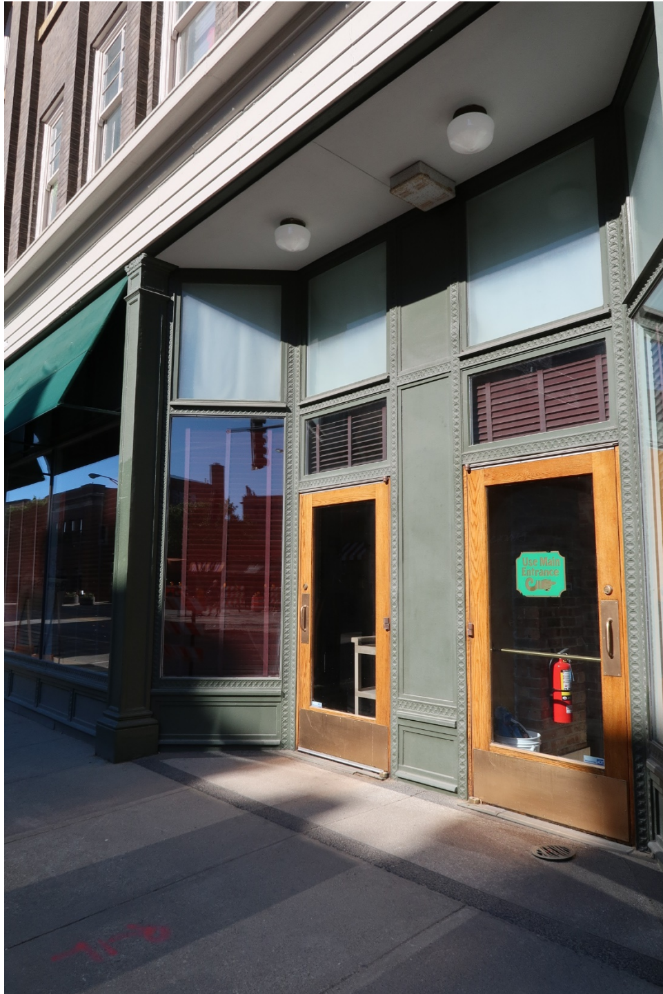
Photo 5: Existing east elevation recessed entry.
