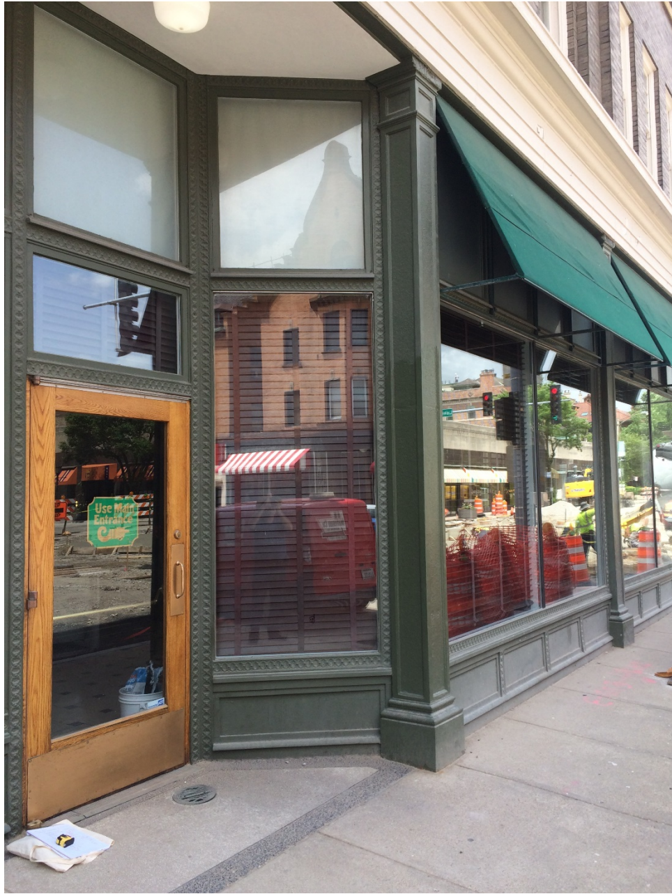
Photo 6: Existing east elevation recessed entry and storefronts.
