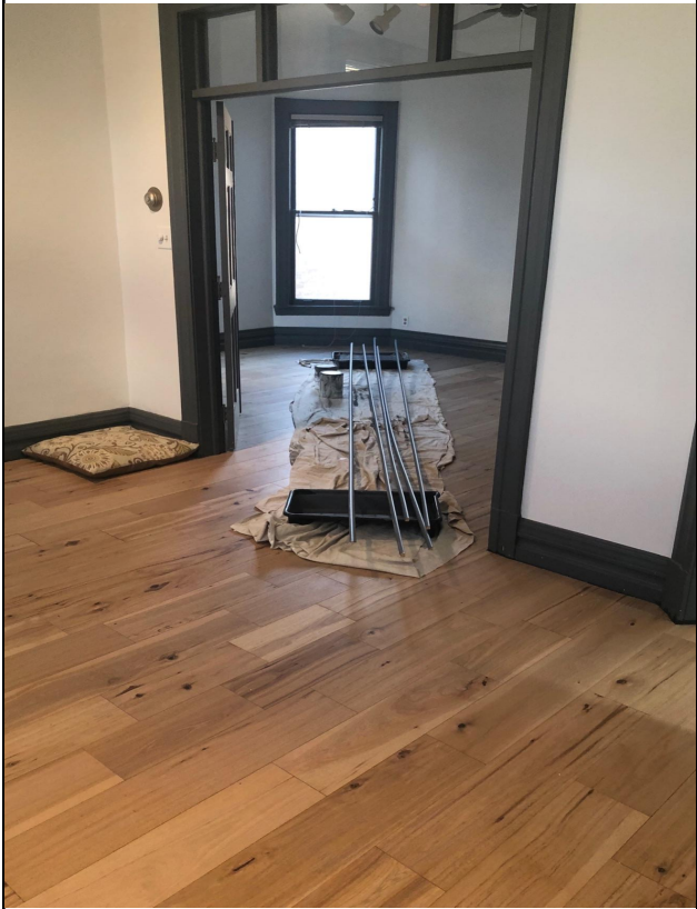
Class Space & Double Door Entrance To Treatment Room 1
