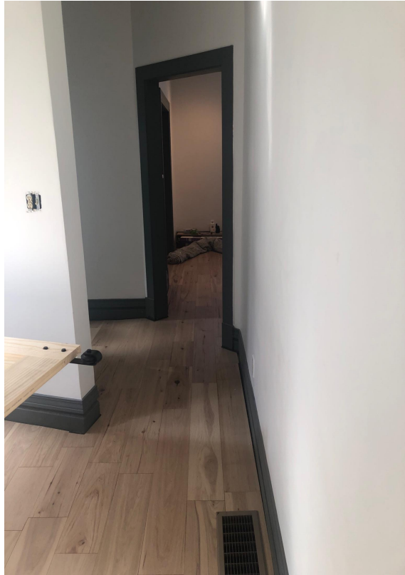
Hallway Looking North into Class Space
