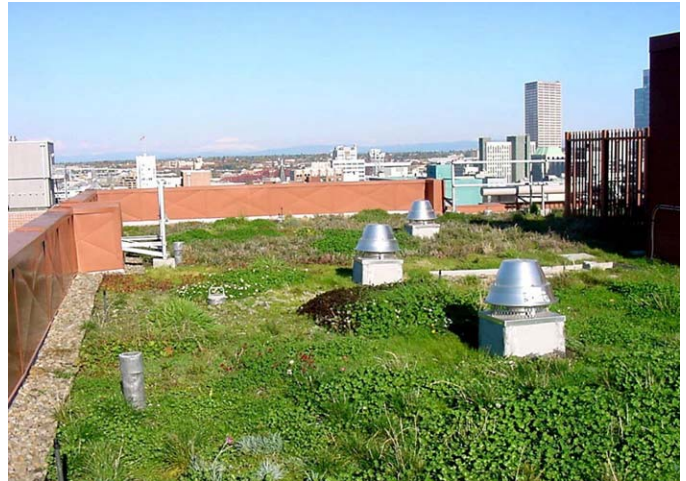
Appropriate Green Roof
