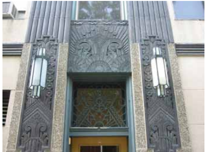
Existing Building Entry at 1103 Westgate
