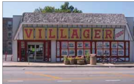
Figure 7.32: Existing Conditions of Storefront Windows in the District
