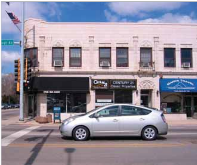
Figure 1.02: Terra Cotta Building Facade at 1142-46 Chicago Avenue
