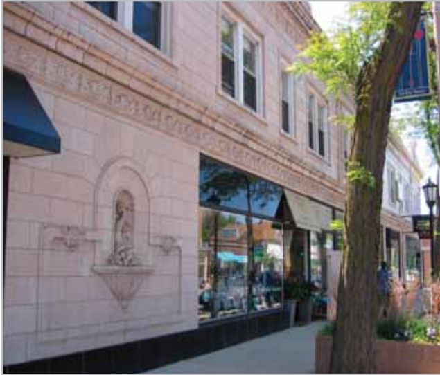
Figure 1.01: Gotsch Building at 1101-13 Chicago Avenue
