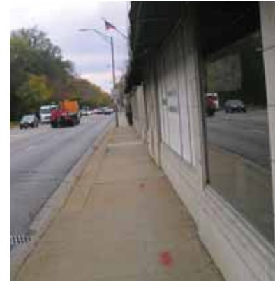
Figure 7.05: Narrow Sidewalk Along Harlem Avenue North of Chicago Avenue
