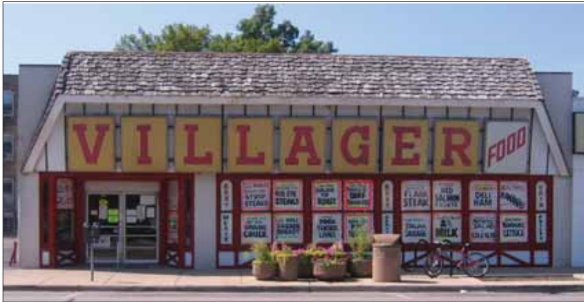
Figure 7.43: Existing Villager Facade Conditions
