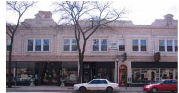
Figure 3.06: Two Story Retail on Chicago Avenue.
