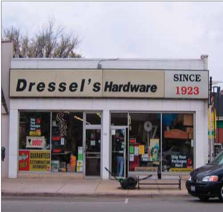
Figure 7.45: Existing Dressel's Hardware Facade Conditions
