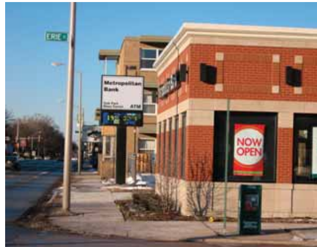
Figure 7.17 New Bank Construction on Erie Street
