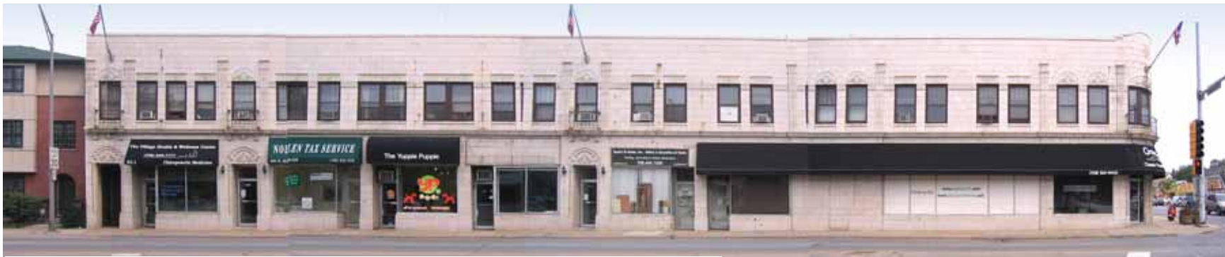
Figure 7.41: Existing Facade - Northeast Corner of Chicago and Harlem Avenues
