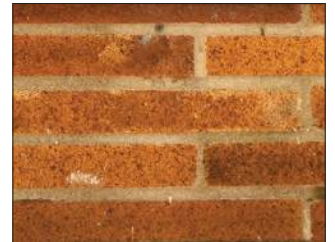
Roman Brick - A hard, dense, fired-clay, regularly shaped building component, with elongated proportions
