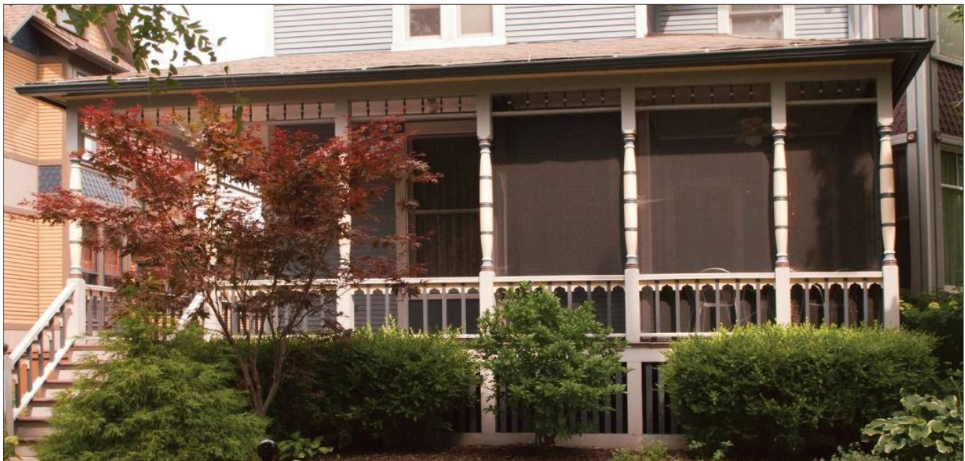
The right side of this porch has been enclosed with insect screens. The screens are installed behind the columns and the balustrade and the supporting structure is not visible from the public right of way.
