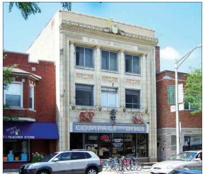
Commercial buildings often used decorative ornament in brick, stone, and terra cotta on the front of the building and common brick on the sides and rear.
