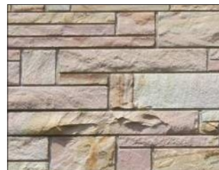
Lannon Stone - A high grade limestone, used as a masonry wall as well as a veneer.
