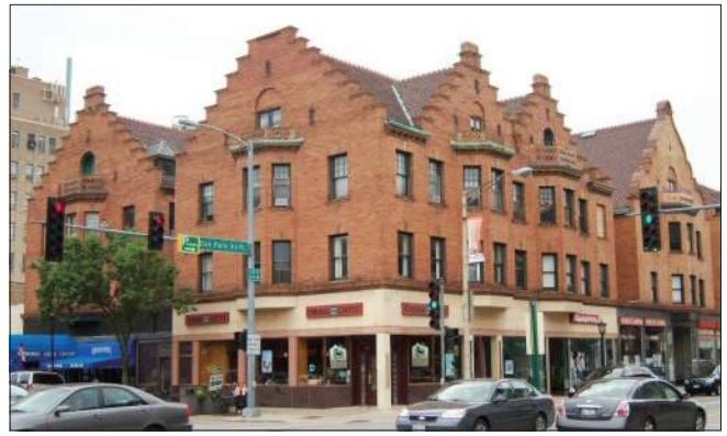
A number of apartment buildings in commercial areas were constructed with commercial spaces on the ground floor.
