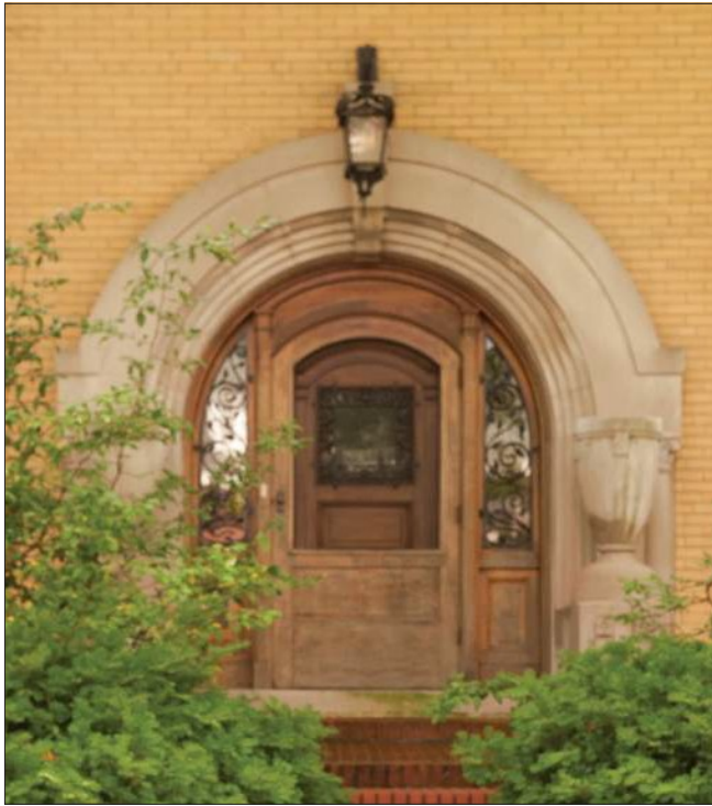
High-style or grand door openings can often include masonry surrounds and decorative sidelights. In this example, the ornate masonry surround is arched and has flanking urns. The paneled, arch-headed wood door is flanked by sidelights and protected by a paneled wood storm door.
