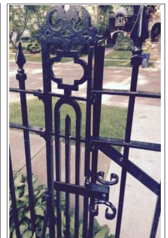
Historic wrought-iron fencing can often be repaired by replacing missing pieces, sanding, powder-coating, and repainting.
