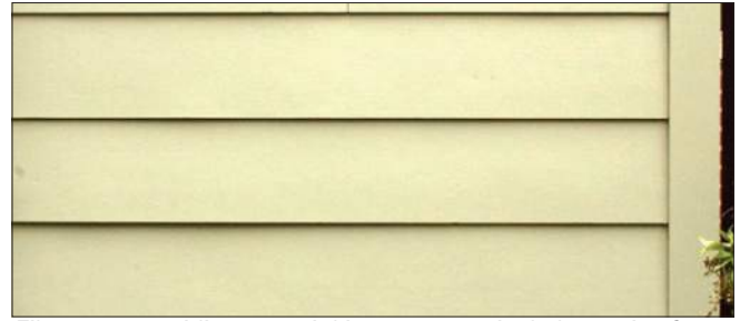
Fiber-cement siding material is an economical alternative for an addition to a historic building. |
