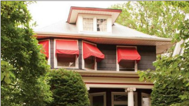
Window awnings can help reduce solar heat gain in warmer months. Awnings should be sized to fit the window opening, and the color and style should be complementary to the house.
