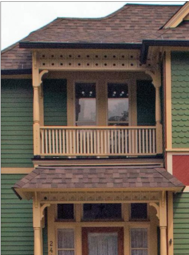
This balcony is located above the entrance and includes similar detailing to the porch below. The balcony is protected by the main roof of the house.
