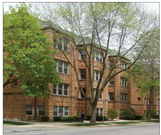
Washington Boulevard has many large-scale apartment and condominium buildings.
