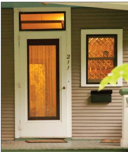
Most Oak Park houses have simple doors, often including glass. A transom window above a door provides ventilation in warmer weather. Also note the leaded glass double-hung window pictured.
