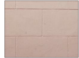
Smooth Finish Stucco - Relatively smooth and flat finish with a plaster appearance.
