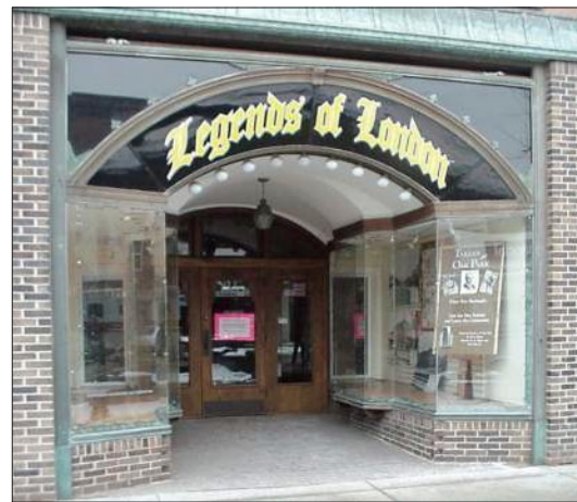
This 1933 Art Deco storefront retains its plate glass display windows, bronze frames, vaulted ceiling, pigmented glass fascia, bronze decorative trim, and entry transom.
