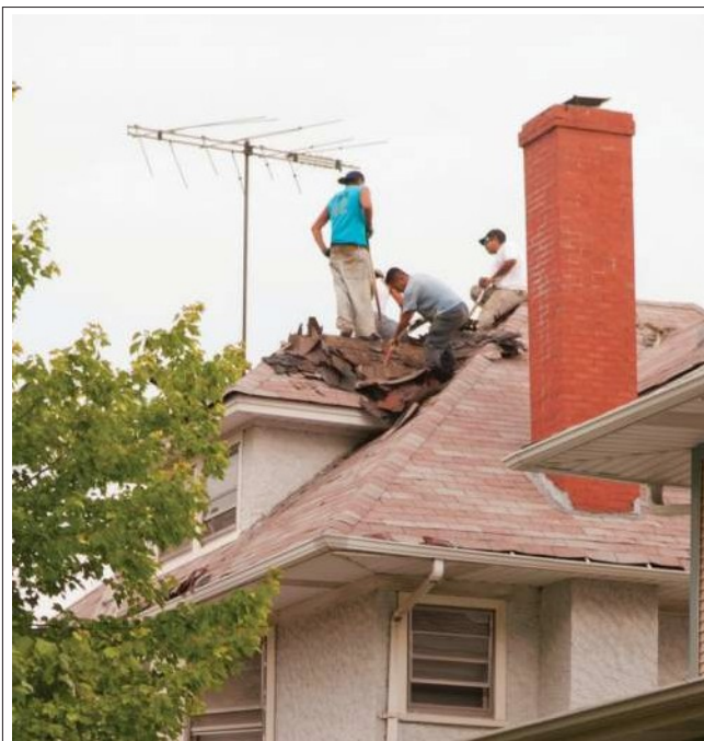
Replacement of exterior building materials such as roofing can maintain a weather-resistant enclosure and protect a home's interior.
