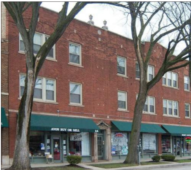
These storefronts are flush with the outside of the building. The entrances include large glazed panels. The doors to the upper level apartments include multiple glazed panels and are topped by a decorative pediment.
