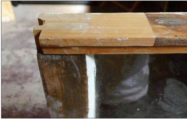
One of the advantages of historic wood windows over modern prefabricated units is reparability. This photo demonstrates a dutchman repair at the corner of a historic wood window. Also note the new glazing putty.
