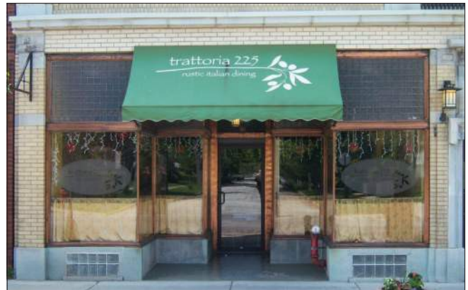
These transom windows are made of Luxfer prism glass, which was invented in 1896 and designed to refract and spread additional light towards the back of the store.
