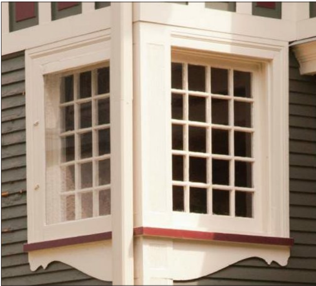
Historic wood windows typically have a three-dimensional quality that does not exist in newer replacement windows. These 20-light corner casement windows have decorative wood surrounds as well as single-light wood storm sash.
