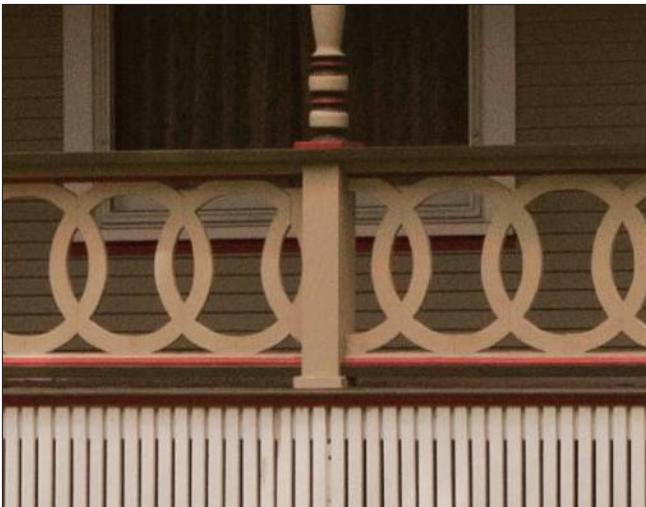
This balustrade is formed of regularly spaced, intersecting circles.
