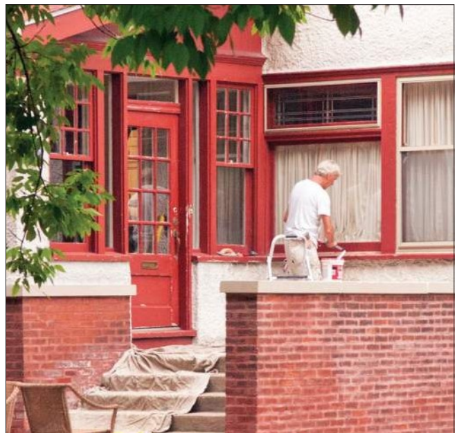
Proper preparation before repainting, including hand scraping, sanding and washing, as well as using quality paint and primer appropriate for the material, will result in a better-quality job. The tarp in the photograph does not meet current EPA requirements for protection of the soil and environment.
