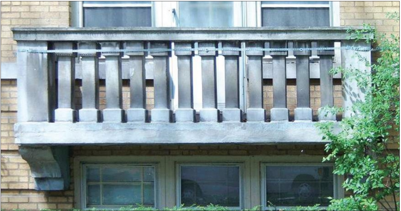
This limestone balcony is supported by brackets flanking the window below and is accessed by a central door. The railing is comprised of square balusters with corner piers.
