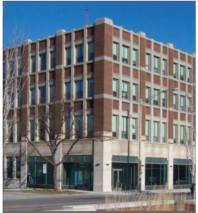
The upper two stories of this building are an addition. The fenestration pattern, materials, and details are compatible with the historic portion of the building.
