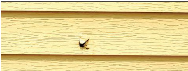
Repair of this puncture requires replacement. Replacement of this aluminum siding is the best way to repair this puncture. A wood-grained texture is generally inappropriate.
