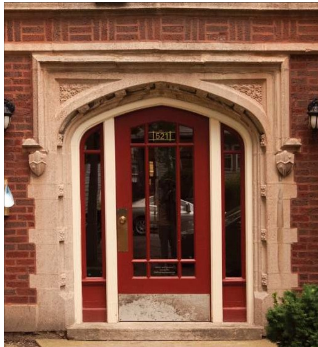
Limestone is often used as a decorative accent element in brick walls and at window and door openings.
