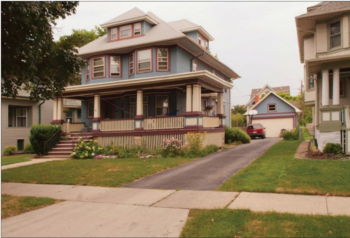
The garage at the rear of the property is accessed by a driveway that runs along the side of the house. The garage includes a gable roof with overhanging eaves and a similar slope as the main house. The exterior of the garage has similar materials to the house, and both share the same paint colors.
