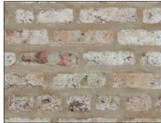
Chicago Common Bond Brick- A hard, dense, fired-clay, regularly shaped building component, sometimes with a glazed surface.
