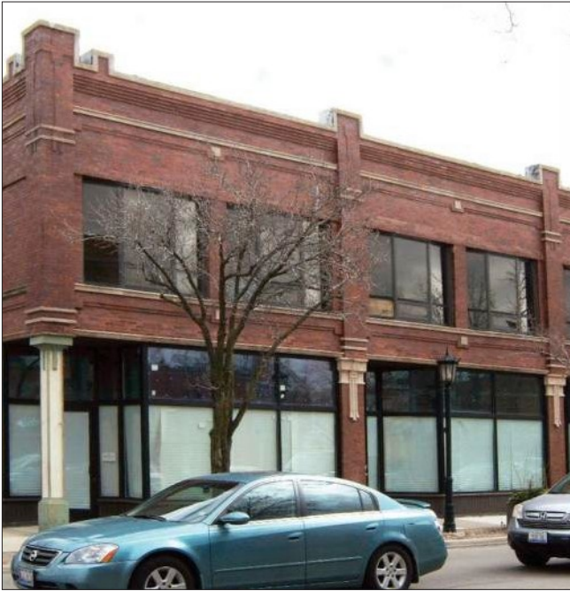
Replacement storefronts often use anodized aluminum. This display window configuration, which includes transom windows above, is located within the original masonry openings.
