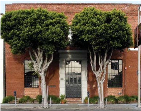
One of a number of historic commercial properties in a historic district renovated by the Ron Kaufman Co., the 1855 Gibb-Sanborn Warehouse, a rare city survivor of the Gold Rush era, is protected by an easement held by San Francisco Architectural Heritage. Photo: ©SF Architectural Heritage.
