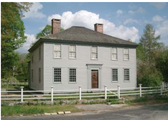
The 1787 Phelps Inn located in North Colebrook, CT is one of several buildings on a 33-acre property protected by a preservation and conservation agreement granted to Historic New England by the late John A. and Nancy Phelps Blum. Courtesy of Historic New England.
