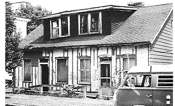
Home in Belleville Historic District before rehabilitation
