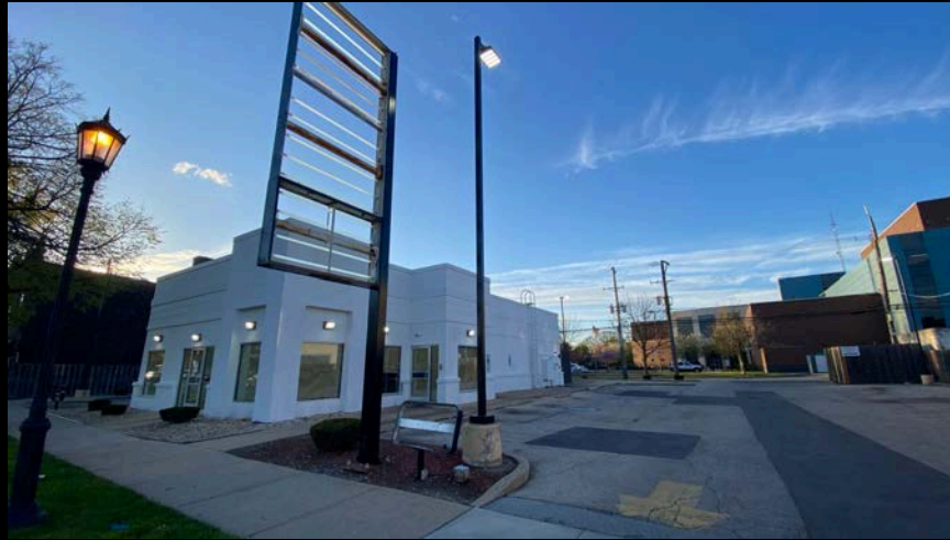
Figure 16: An unoccupied commercial building on Madison. The multiple, unshielded, high-intensity LED wall-packs and parking lot lights are on during the day and are exceedingly bright at night with no clear purpose.
