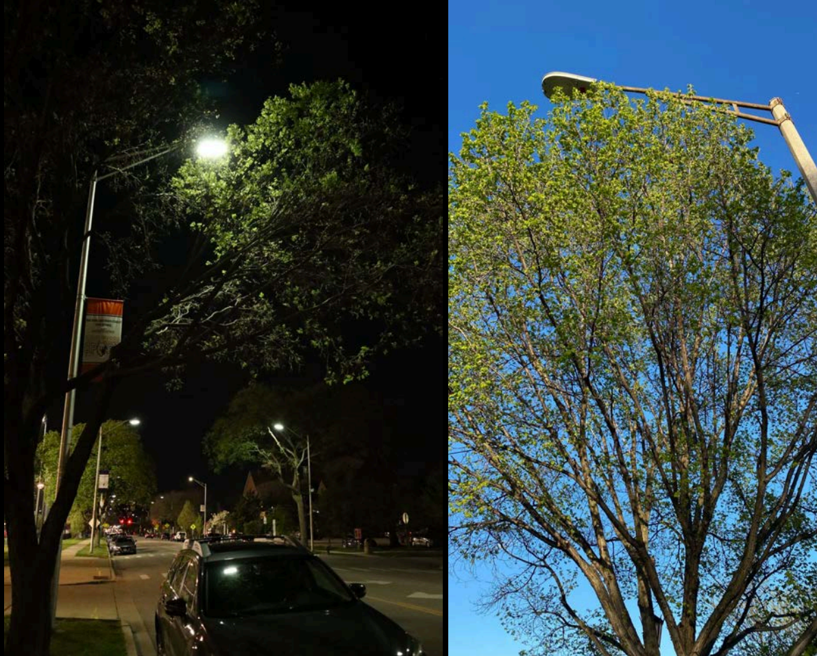
Figure 7: Examples of lights obstructed by trees rendering them virtually ineffective and an ecological hazard.
