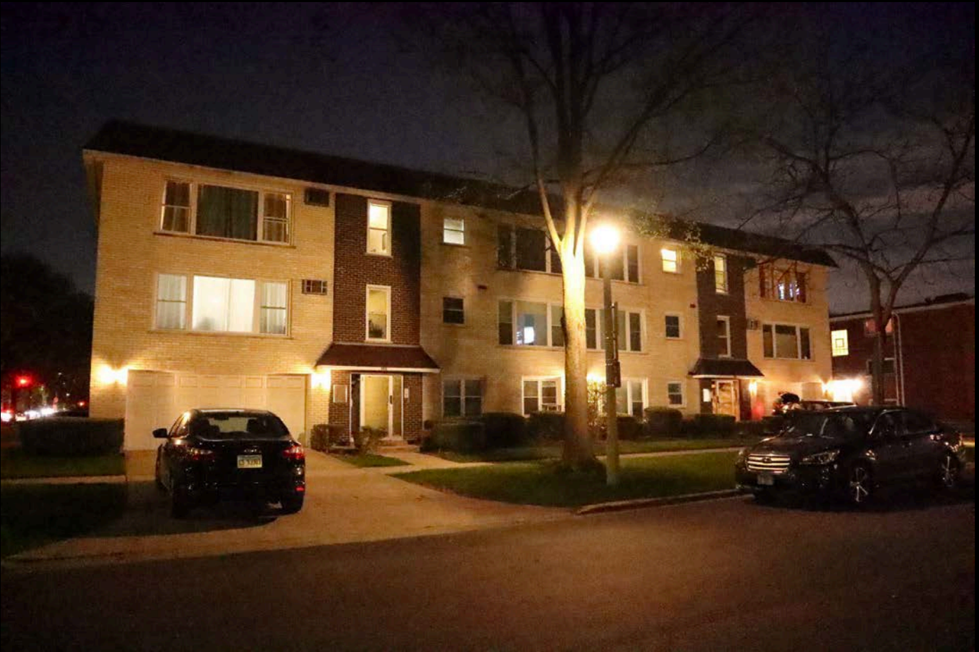
Figure 9: Examples of undesirable light trespass from street lights in residential areas. (Top Left) High level light spill on a residence on Fillmore from a “full-cutoff” LED street light. (Top Right) House windows illuminated by King Arthur street light. (Bottom) Excessive light trespass on residential windows from a King Arthur fixture on Wesley.
