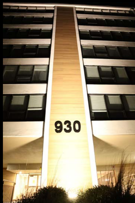
Figure 15: Additional examples of uncontrolled uplighting at a bank building (top left), 700 block of Lake St. (top right), apartments (middle) and 900 block of North Blvd. Since the lights seen in the middle photos are at ground level, they create direct glare to motorists (middle left) and cause high levels of light trespass into trees and residential windows.
