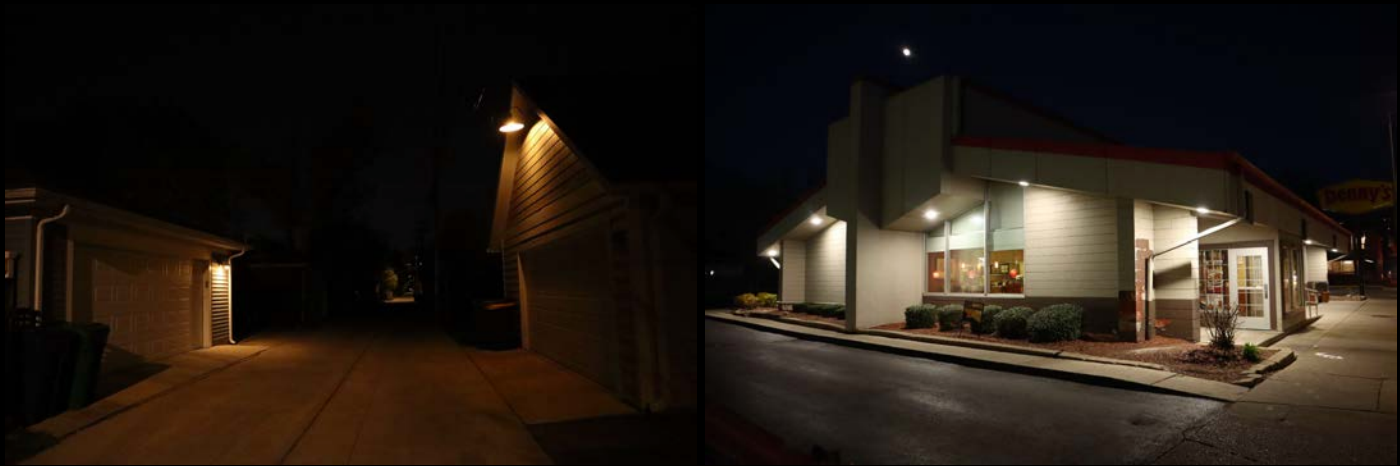
Figure 18: Examples of well applied lighting. A good example of the use of private lighting used to illuminate the garage and alley (left). The light is at an appropriate level, shielded and a warm color temperature. [Note: the addition of motion sensors could improve the effectiveness and efficiency of this lighting]. Good example of commercial lighting (right). The under canopy lighting eliminates all uplight. The recessed can lights eliminate nearly all glare. The establishment remains well lit.
