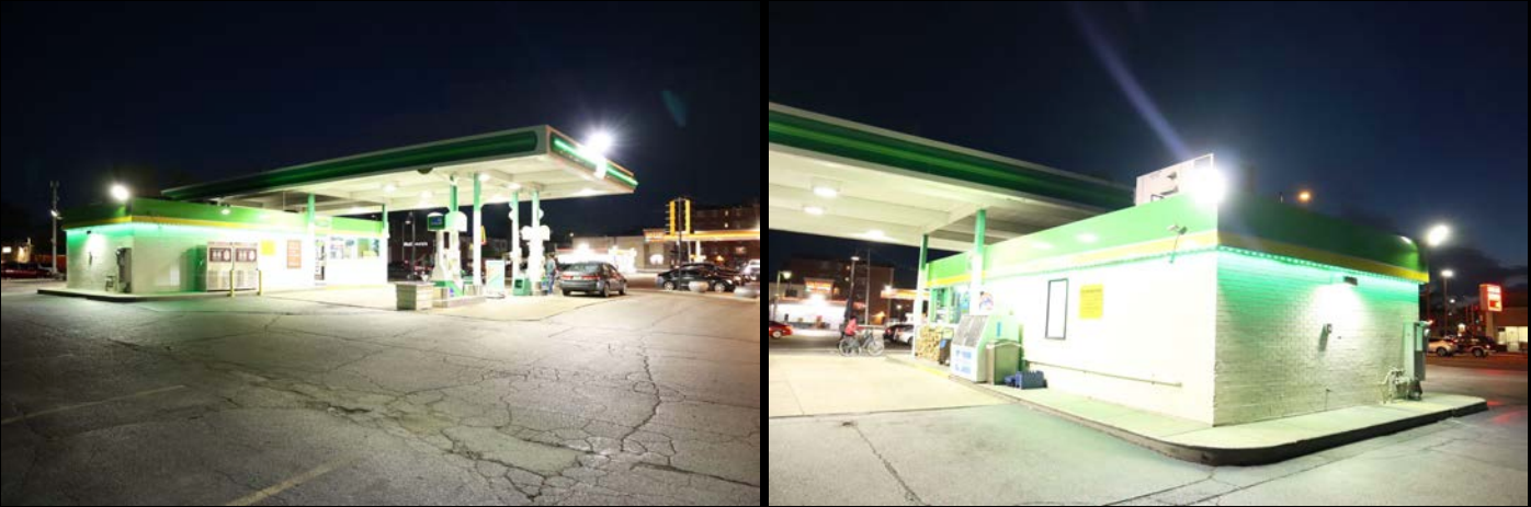
Figure 12: Gas station on Roosevelt. The use of high lumen, 5500K, LED flat panel lights inappropriately tilted above 90 deg generates dangerous amounts of glare and trespass. The excessive glare - at a busy intersection - can create visibility issues for drivers.
