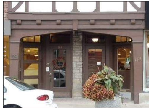
This alcove encompasses two storefront entrances and is capped by a Tudor Revival style cornice.
