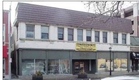
The Boulevard Arcade Building is a Landmark that used the Cook County Class L tax incentive to restore the façade and interior for office use.
