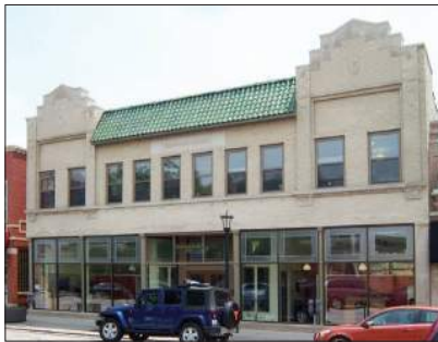
This commercial building includes the building name on the transom window above the entrance and engraved in stone on the second floor.
