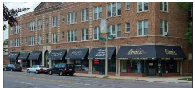
The awnings are located within each of the building's bays, providing a unifying element for the building.
