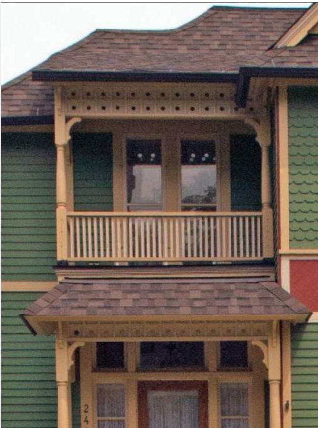
This balcony is located above the entrance and includes similar detailing to the porch below. The balcony is protected by the main roof of the house.
