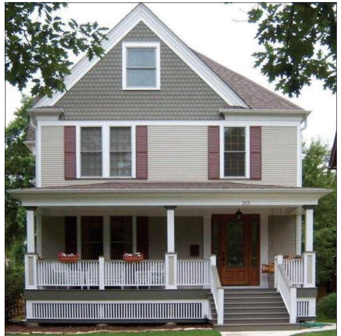
The original porch was missing and replaced with a compatible style, including scale and setback.
