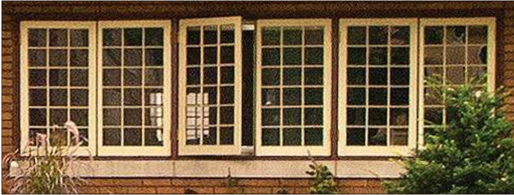
This band of three paired 18-light, wood casement windows have true divided lite muntins. The windows provide interior illumination and allow for ventilation.
