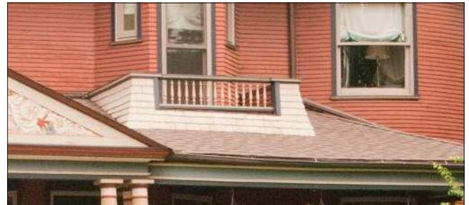
A balcony is a platform enclosed by a railing that projects from an upper floor of a building.
