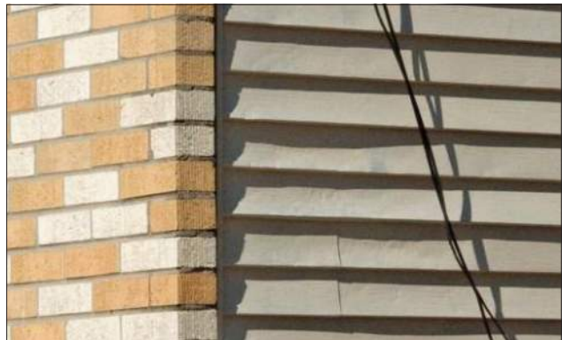
The left wall of this wood-framed house has been covered with brick veneer. The addition to the right has been covered with vinyl siding. Both are inappropriate materials and should not be used on historic buildings.
