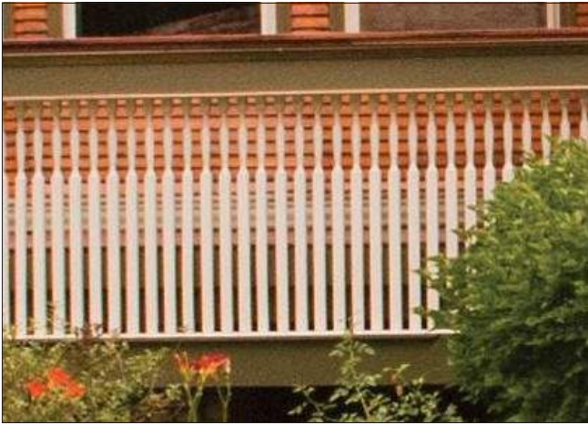
Most balusters in Oak Park are square or turned wood. This example includes a turned detail at the top of each baluster.
